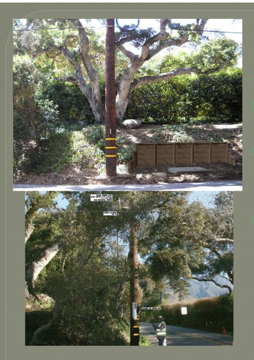
Vault requires 4' h x 14' l retaining wall Ground cover removal required
