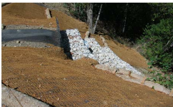
Stagecoach Rd MP 3.5 Gabion Outlet Drainage
