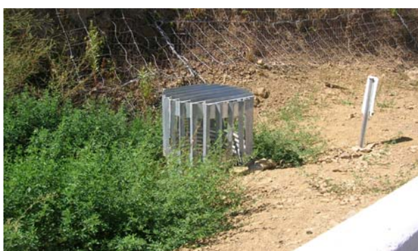
Stagecoach Rd MP 3.5 Inlet Debris Rack Riser
