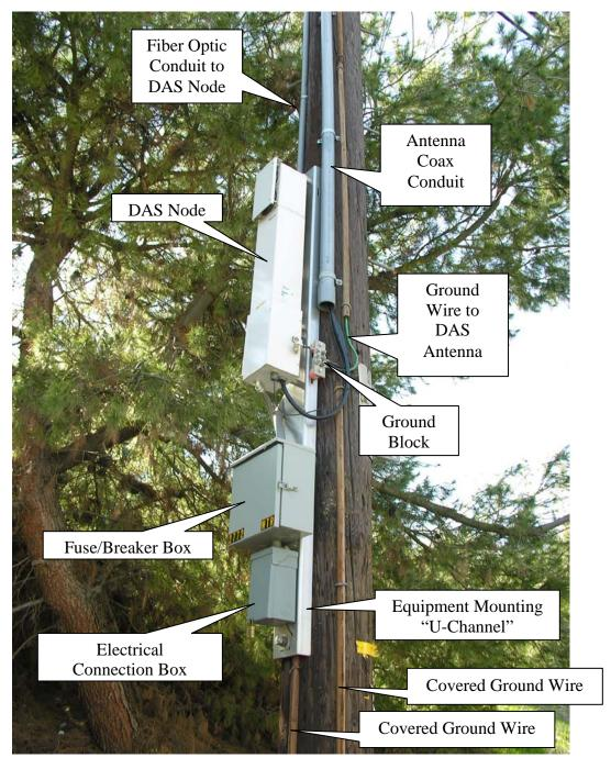
Figure 1: NextG Node Installed on a Utility Pole in Rolling Hills Estates, California.
