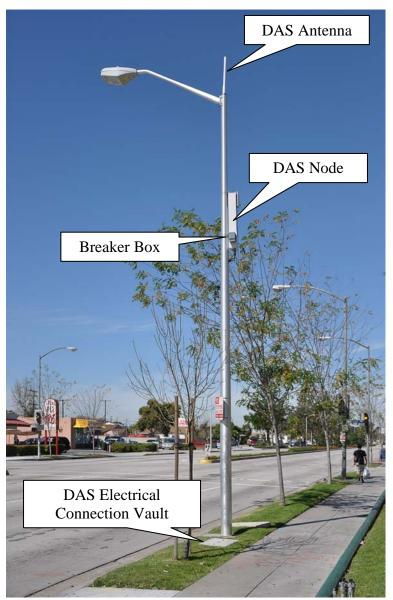
Figure 4: NextG Node Installed on a Street Light in Norwalk, California
