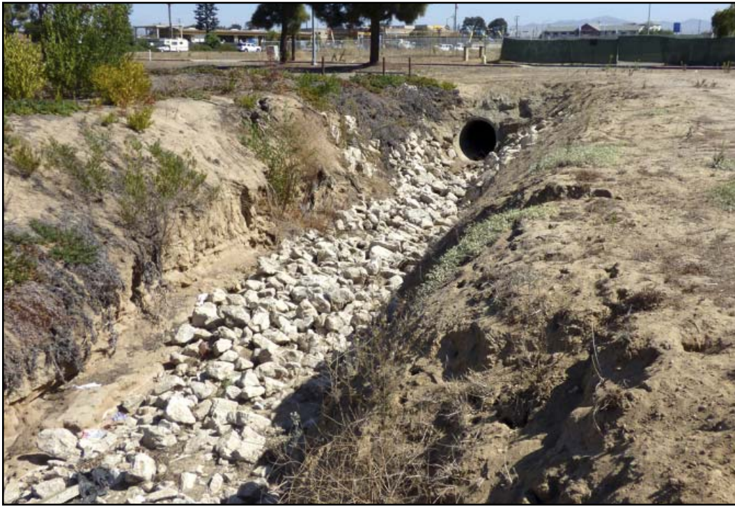
PHOTOGRAPH 5 Views of SMAD Inlet Looking South Towards Staging Area
