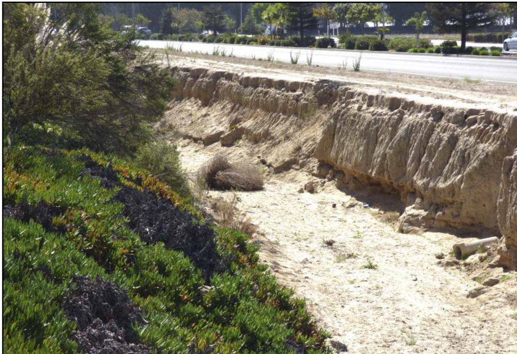
PHOTOGRAPH 2 Views of Erosion of Bank at SMAD Curve
