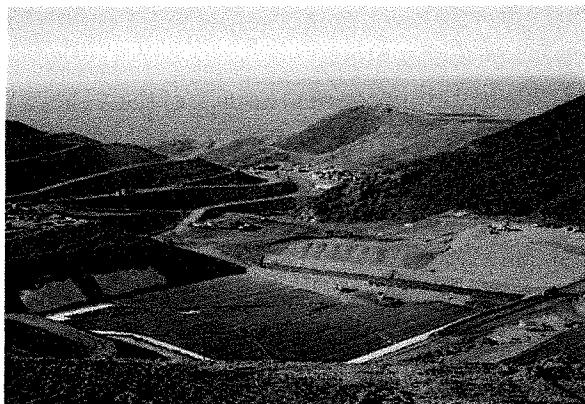
Liner system installation of Phase IIIB GWPS Project
