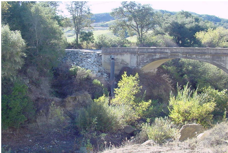
Photo: Existing Bridge 51C-113
