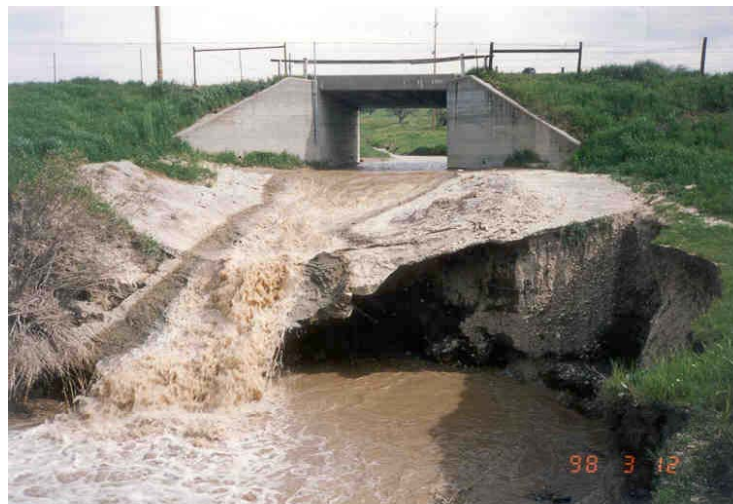
Photo: Existing Zaca Station Road Bridge 51C-087 and channel conditions
