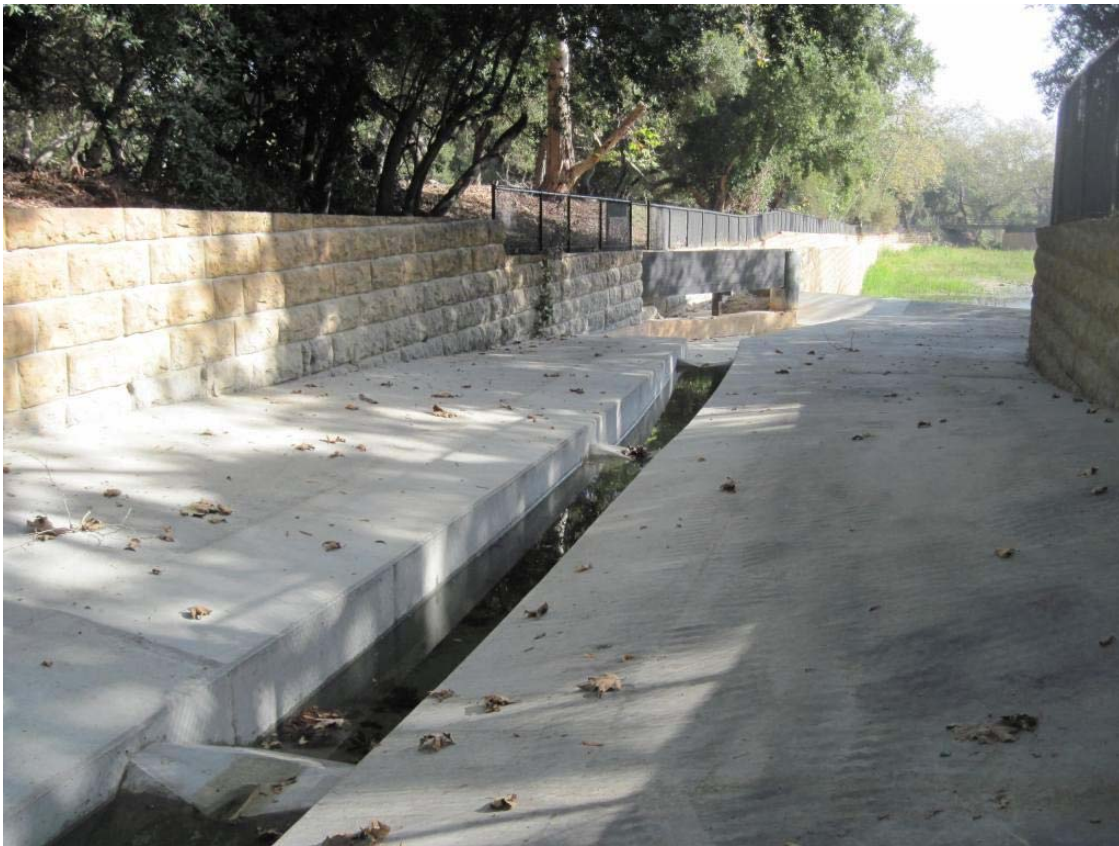
Montecito Creek Fish Passage Project Completion
