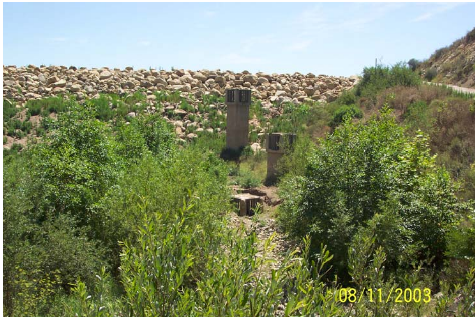
Santa Monica Debris Basin Towers (A, B, and C)
