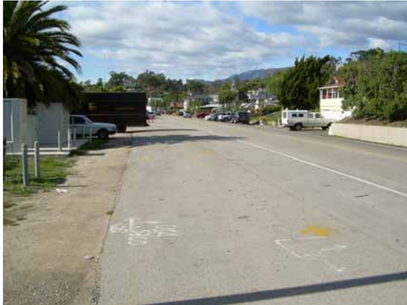
Lillie Avenue (preconstruction)
