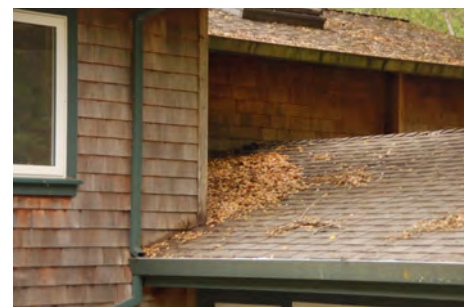
Replacing siding “locally,” in areas where it meets the roof on a complex roof design, such as that shown here, would be more affordable than “global” replacement. Source: Stephen L. Quarles
