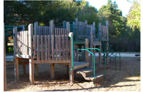
A wood play structure. Note the larger wood members in this play structure. The bark mulch used for the surfacing material pose a bigger threat in terms of ease of ignition from an ember exposure. Source: Stephen L. Quarles
