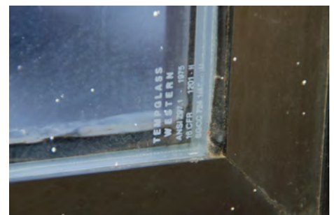
Etched “bug” in the corner of a window indicates that the window glass is tempered. Source: Stephen L. Quarles
