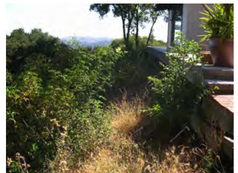
A small deck on a house located at the top of the slope. Source: Stephen L. Quarles
