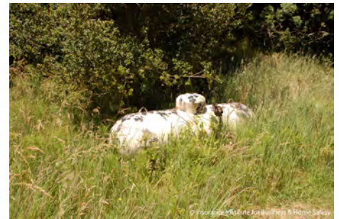
Poor defensible space near a propane tank. Ignition of this vegetation would provide a longer exposure to heat. Depending on level of fuel in the tank, an explosion would be possible under this scenario.
