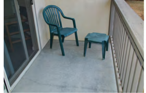
A deck with a lightweight concrete (noncombustible) walking surface. Source: firecenter.berkeley.edu/bwmg/decks-1.html
