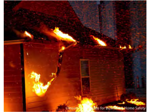
Wind-blown embers ignited debris in a gutter. Photo shows detaching vinyl gutter (left side) and attached metal gutter (right side).
