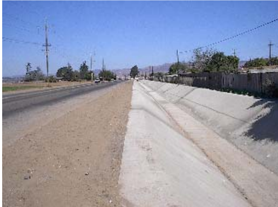
Blosser Channel Improvement Project Completion
