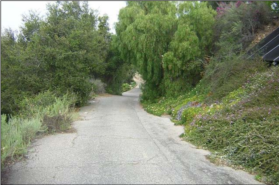
Lower portion of San Antonio Creek Road looking down the road east of Fee Residence. The road narrows to approximately 13 feet in width in this section. Roadside vegetation is encroaching into the travel lanes.
