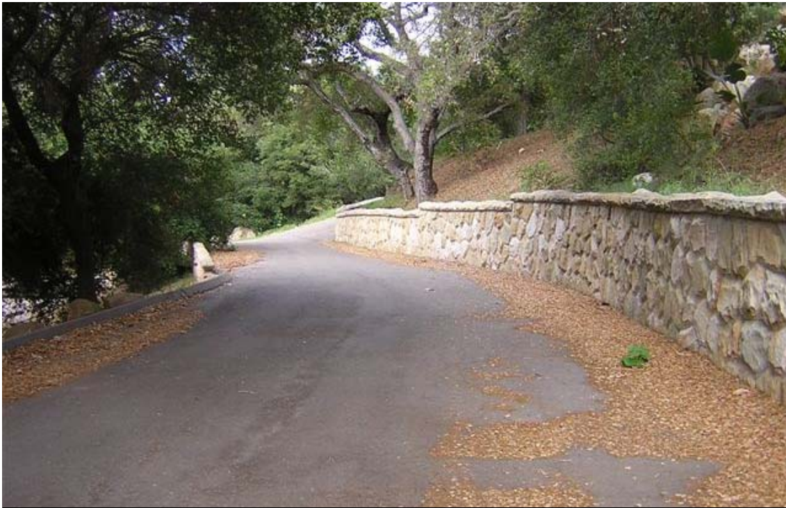
Lower portion of San Antonio Creek Road adjacent to Fee Residence. The road is approximately 22 to 24 feet in width in this section. The retaining wall was constructed in 2007 to restore adequate road width.
