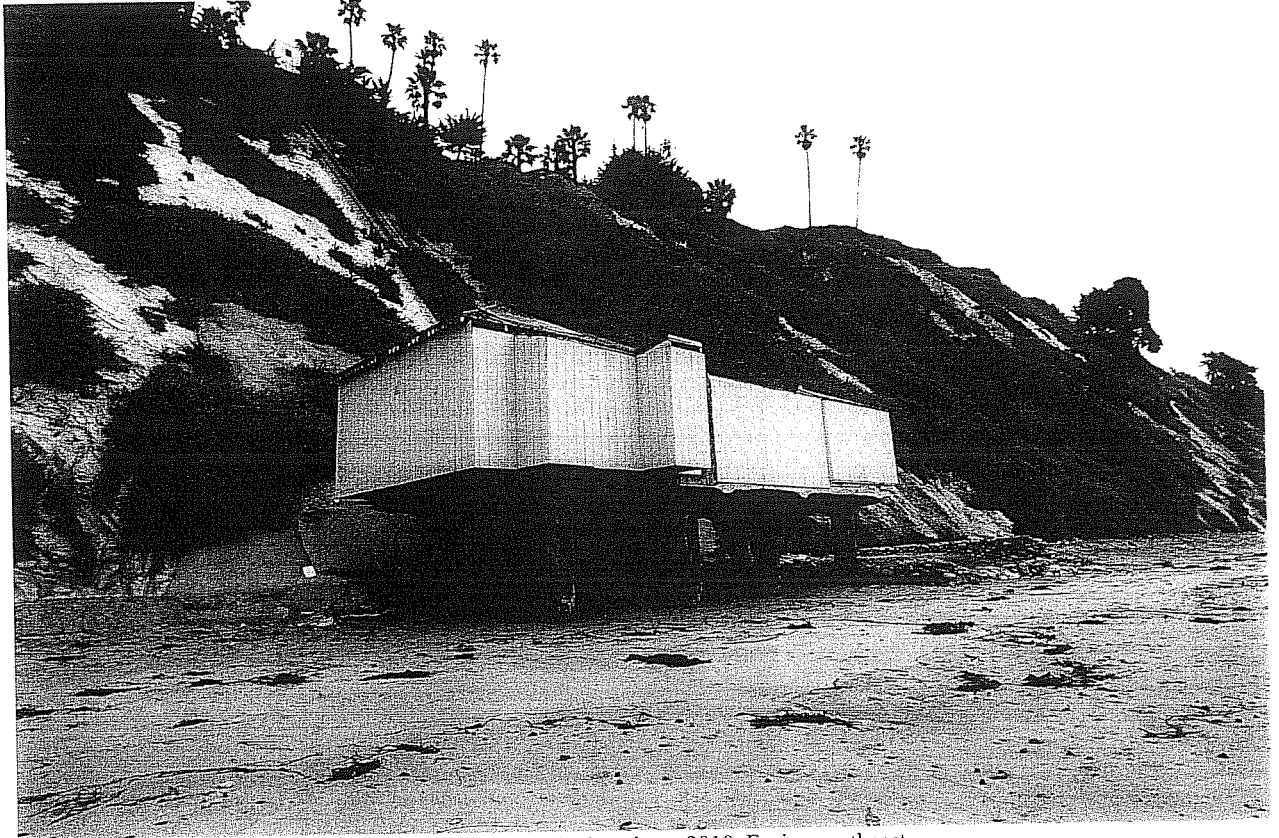
Beach cabana, west and south elevations, 2010. Facing northeast
