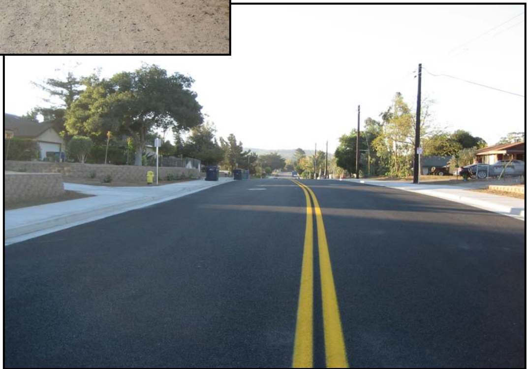
Hummel Drive After Project Completion
