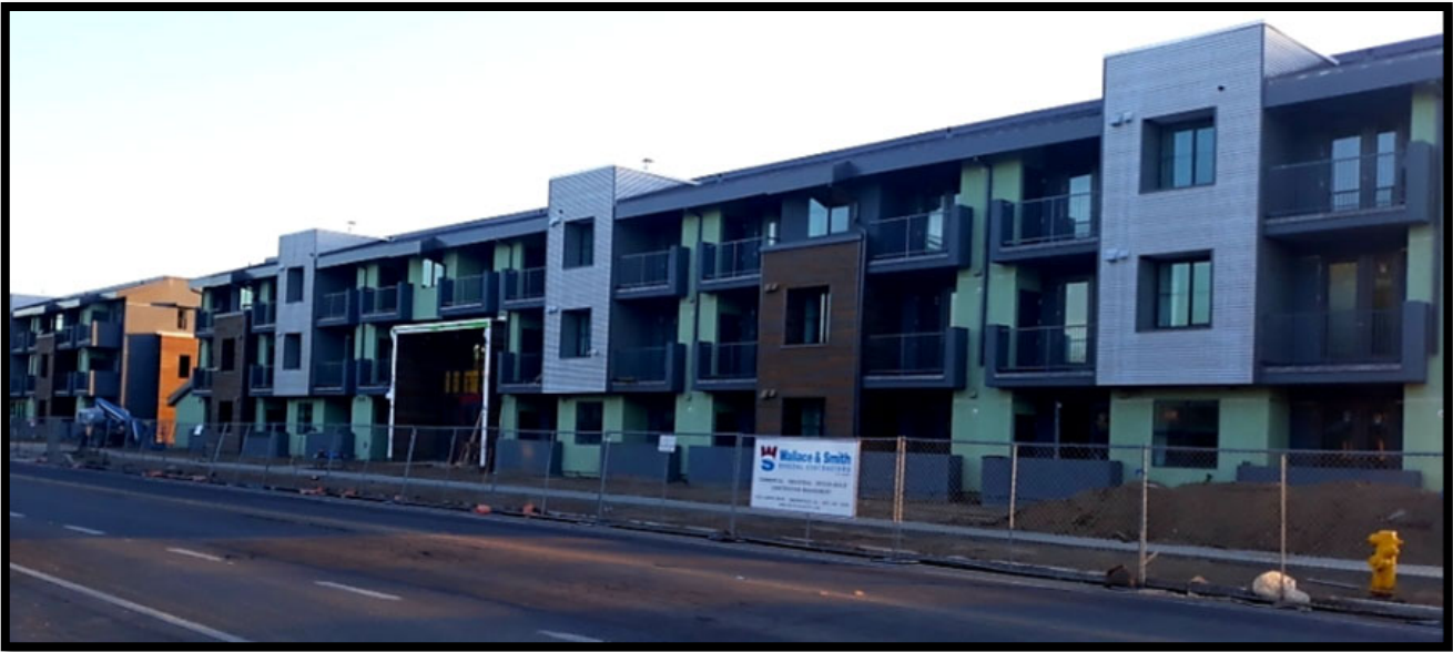
Picture of Residences at Depot St. during construction, photo provided by Prop 63 funded Help@Hand team
