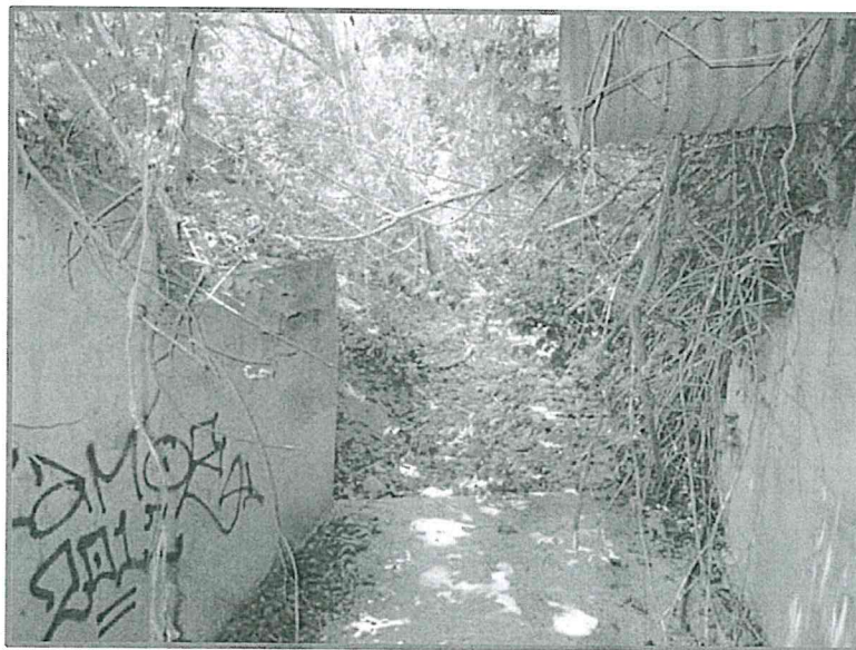
Photo 2: Inlet of existing channel, north side of Hollister Ave
