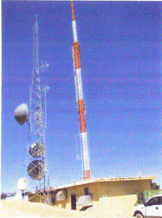
Facility 2 south - Cowles California Media
