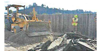
Digouts, Striping, Marking, and Curb Painting
