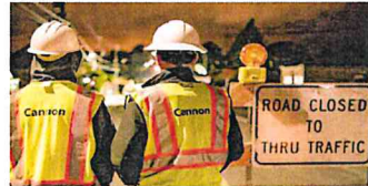
Pavement Rehabilitation and Full Depth Reclamation
