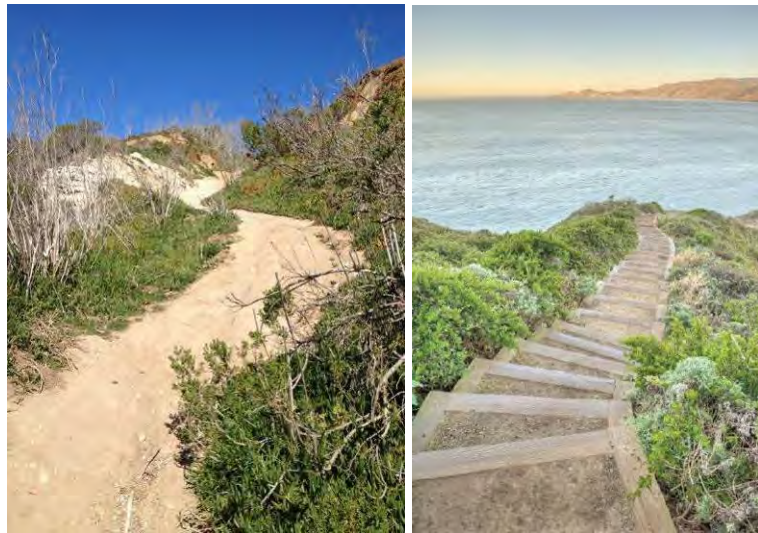
Beach Access Point F: Under the proposed Project, safe beach access would be provided by a stairway, which would be constructed at specifications that meet the natural surroundings of Ellwood Mesa. The stairway (right) would also serve as a permanent solution to erosion and gullying along Beach Access F.
