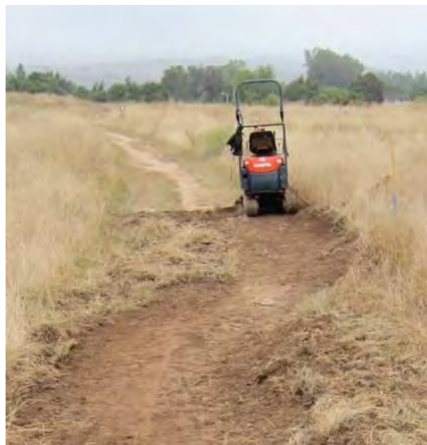
Limited heavy construction equipment would be required for recontouring of the trail surface (such as the equipment shown above, used for minimal trail disturbance at Lake Los Carneros). (Photograph courtesy of Ray Ford)
