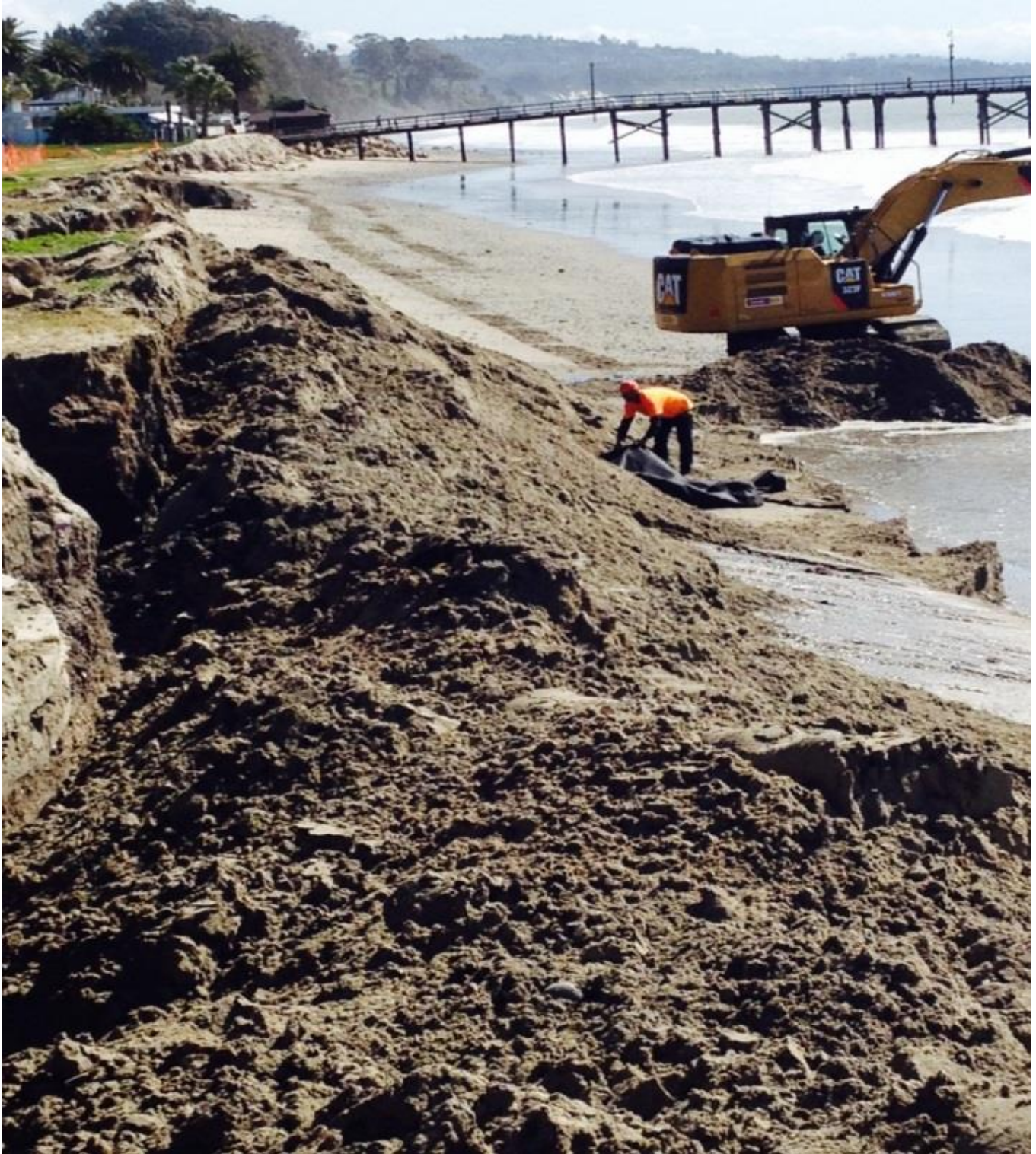
Soil backfill and vertical fabric filter layer install (Mar 14)
