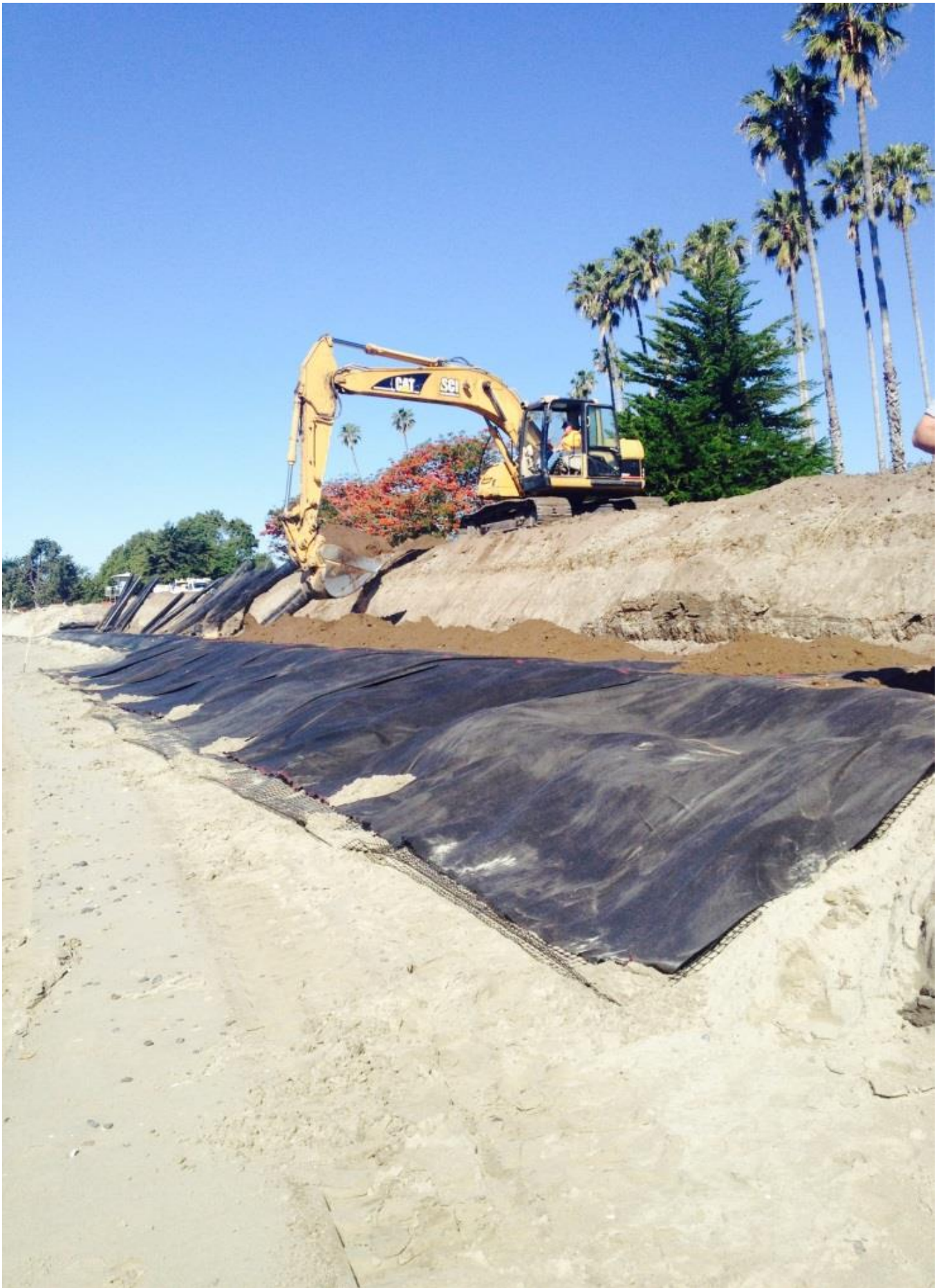
Layer of filter fabric being filled with earth (Mar 31)
