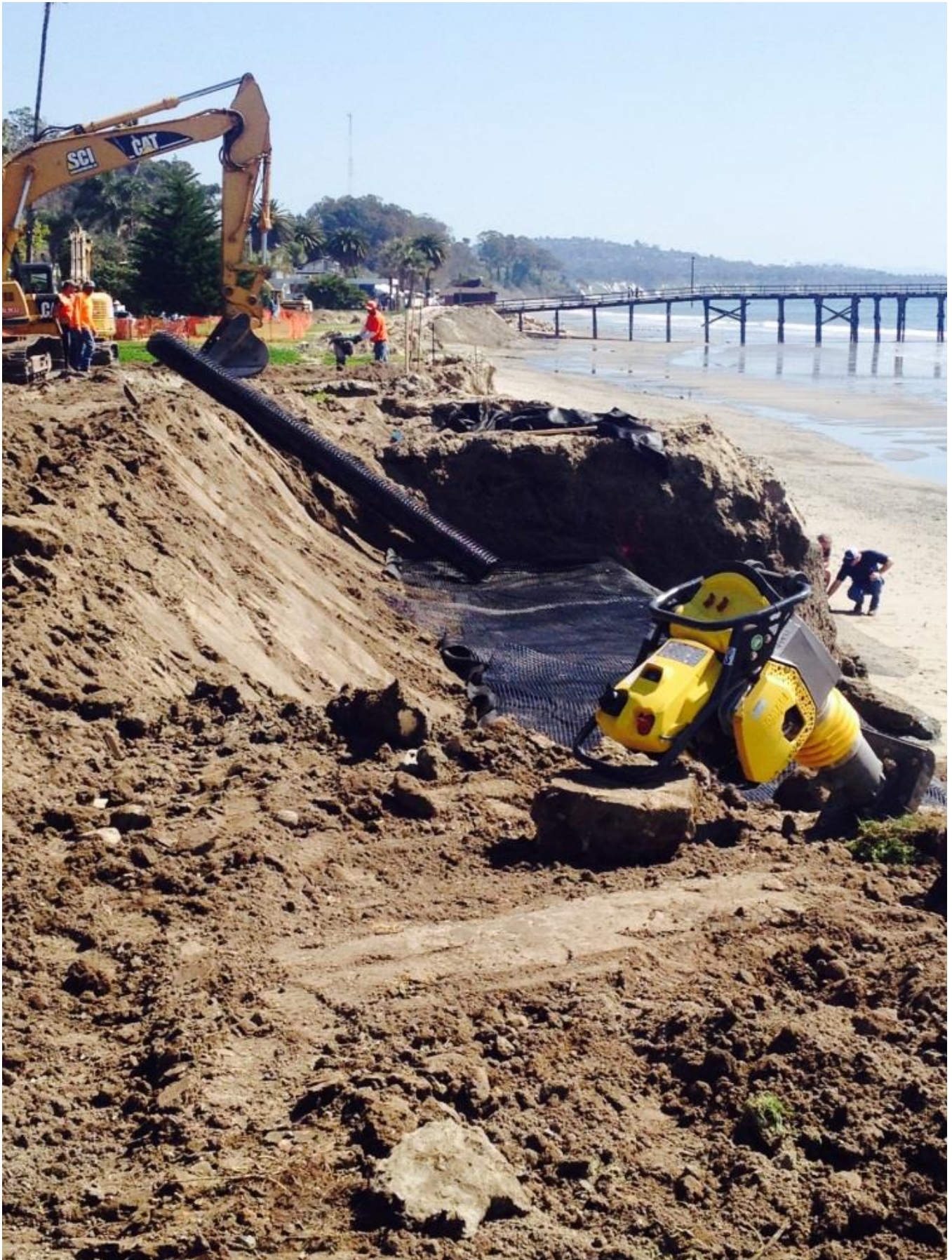
Layer of filter fabric laid open (Mar 17)
