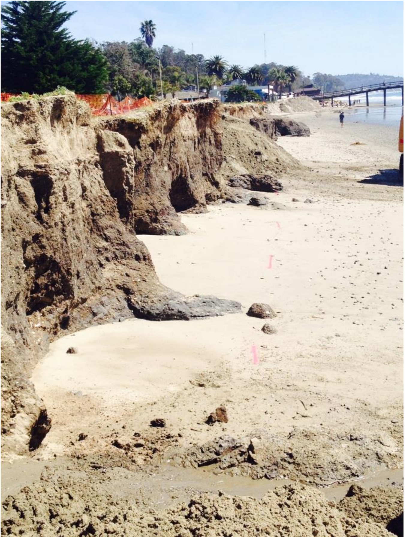
Soil fill line (still 5 to 10 feet landward of land edge prior to Dec 2015)
