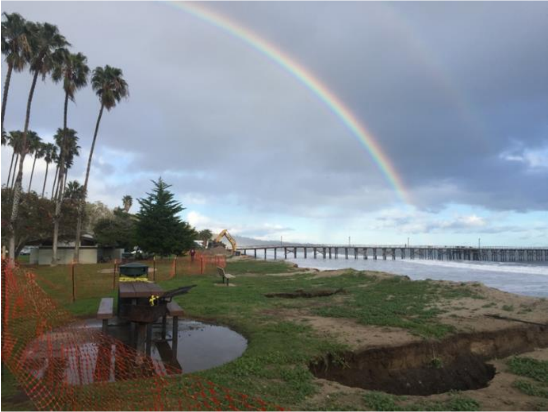
Sinkholes and erosion aspect east (Mar 7)
