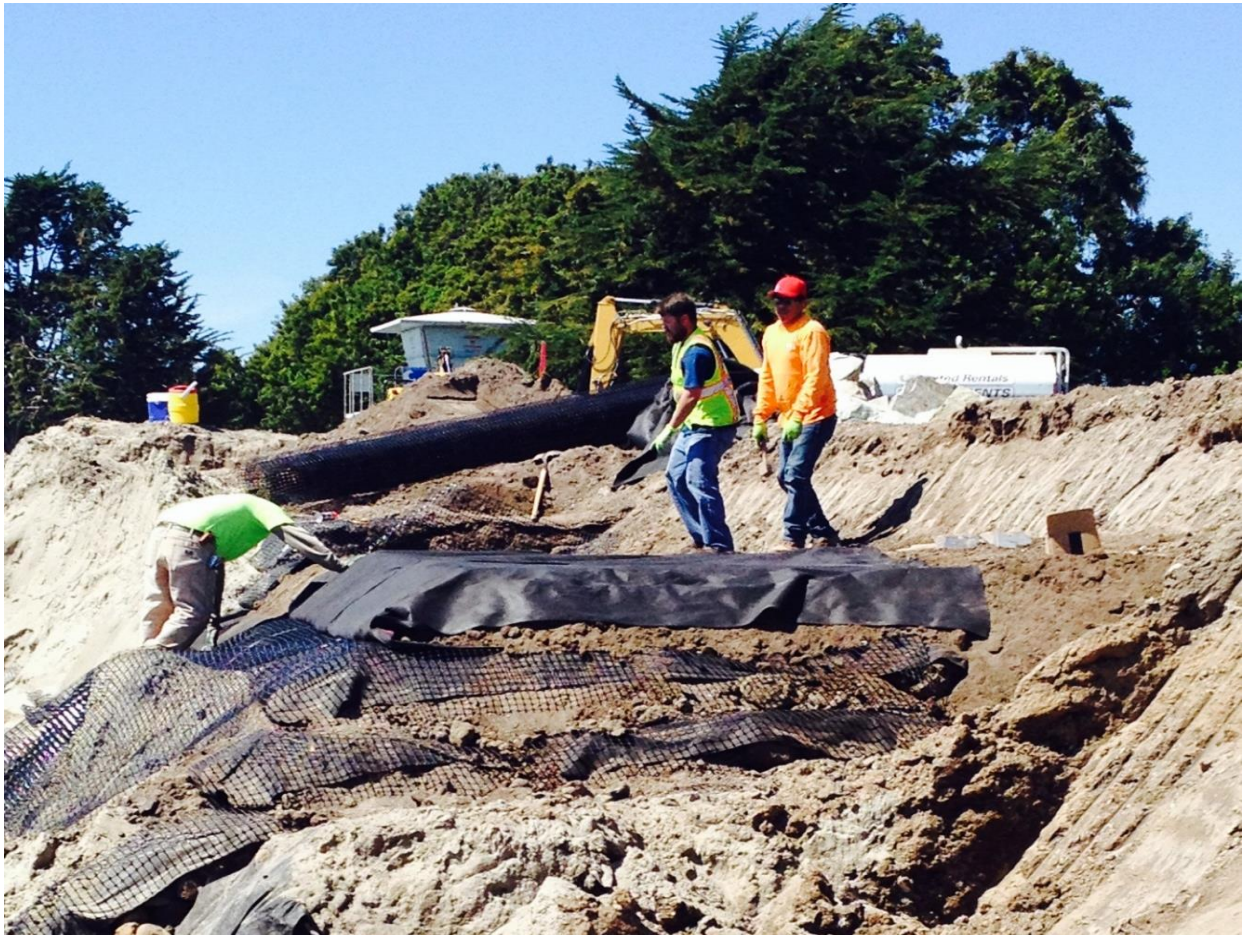
Layered and filled filter fabric cells (Mar 23)
