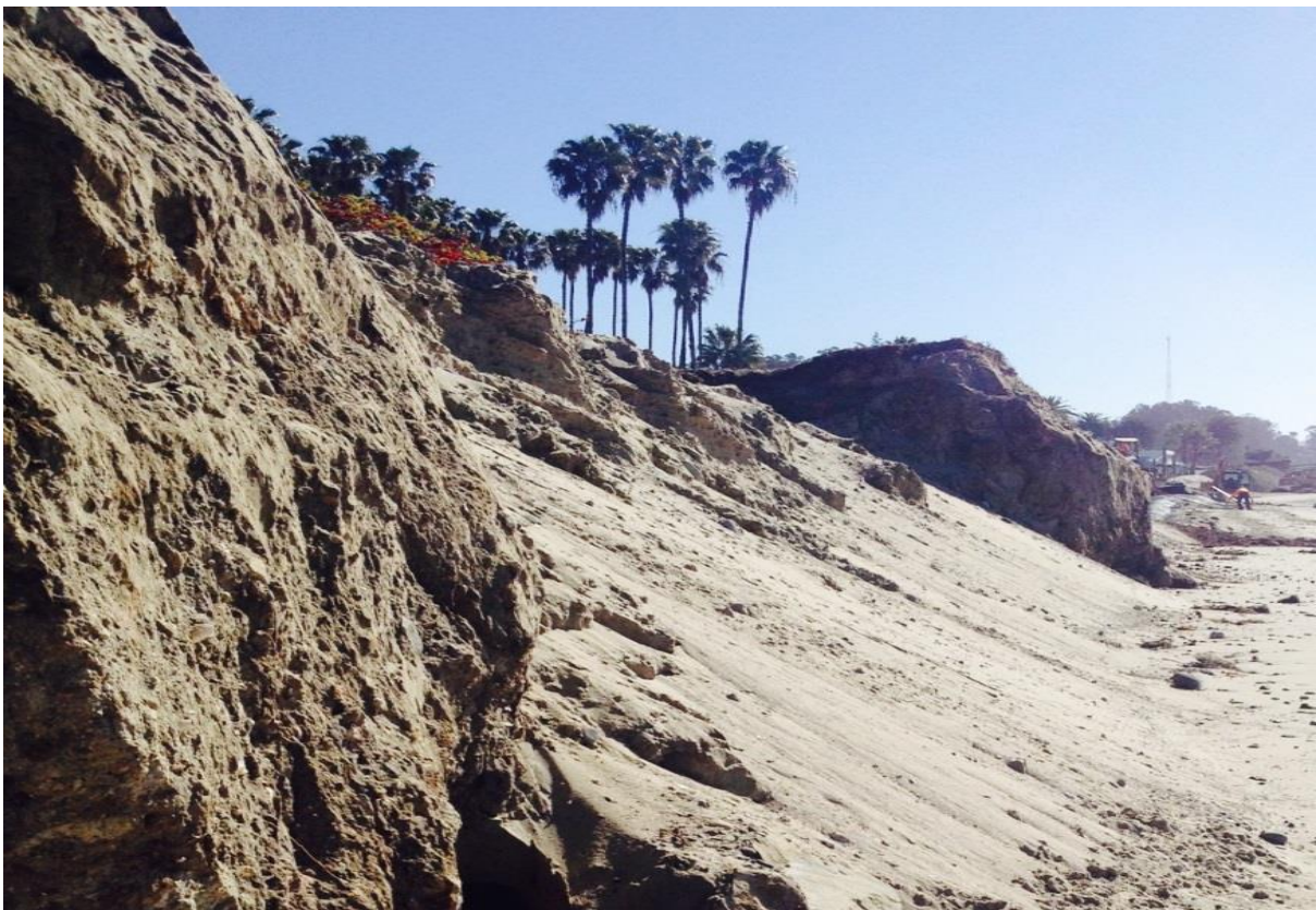
Repaired area facing east (Mar 31)
