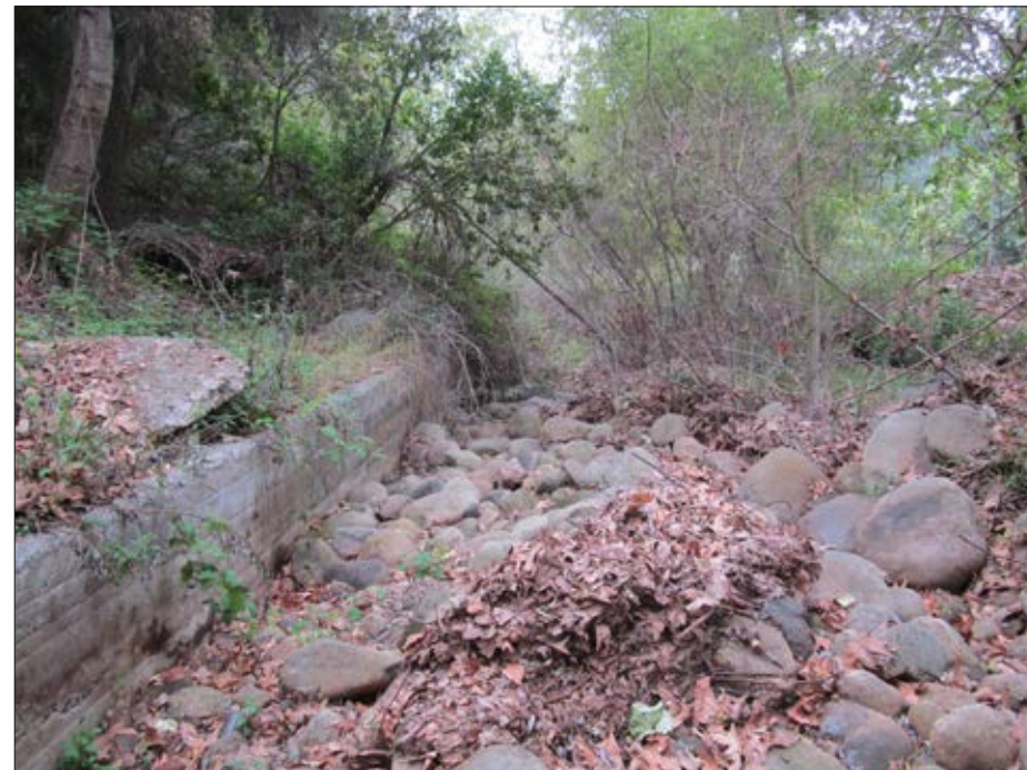
Photo 5: View of paved low water crossing & grade control crossing looking south
