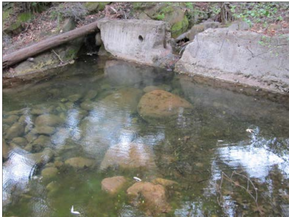
Photo 4: Detail view of old flood gate and wall structure looking north
