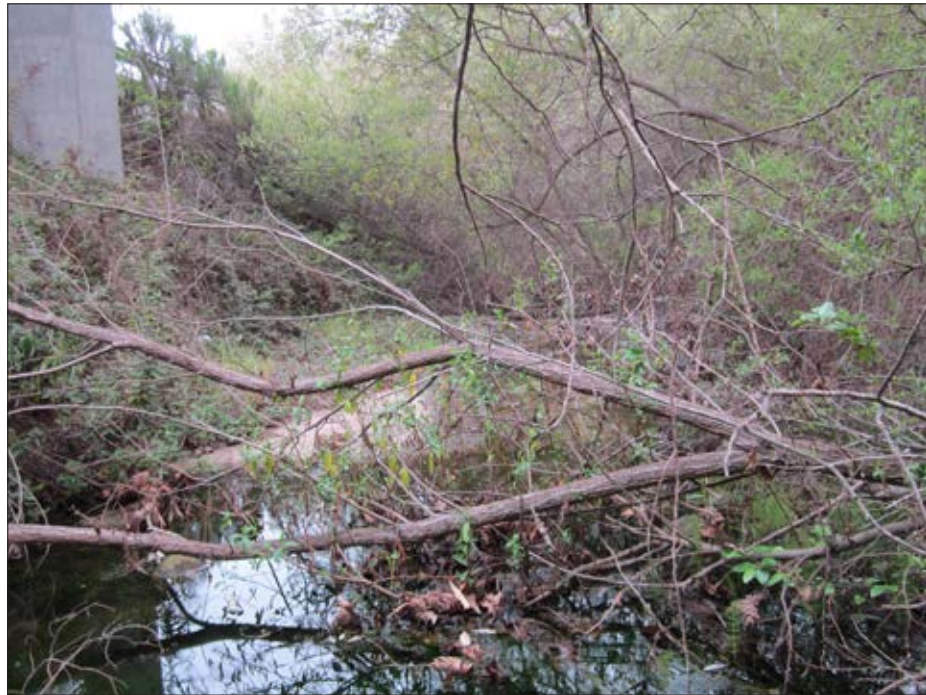
Photo 4: View looking south along creek to old concrete paving under bridge
