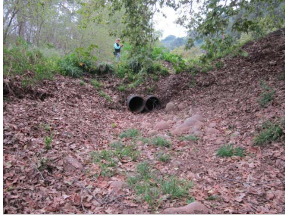
Photo 2: View of dual culverts at culvert crossing looking south
