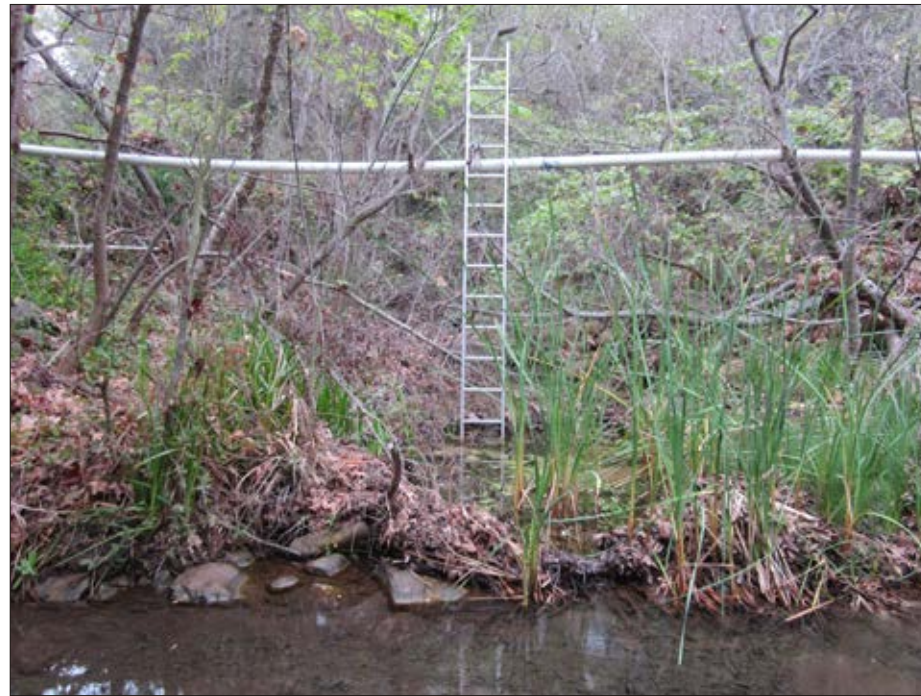
Photo 2: View of unpaved low water crossing looking upstream (north)
