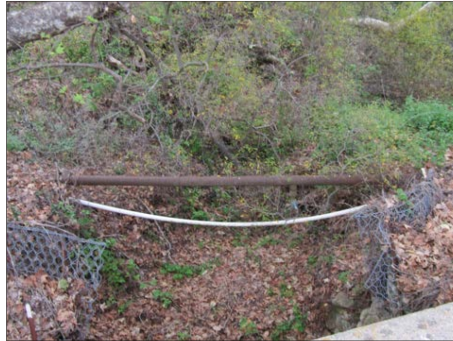
Photo 2: View of secondary drainage downstream of agriculture drain structure/culvert
