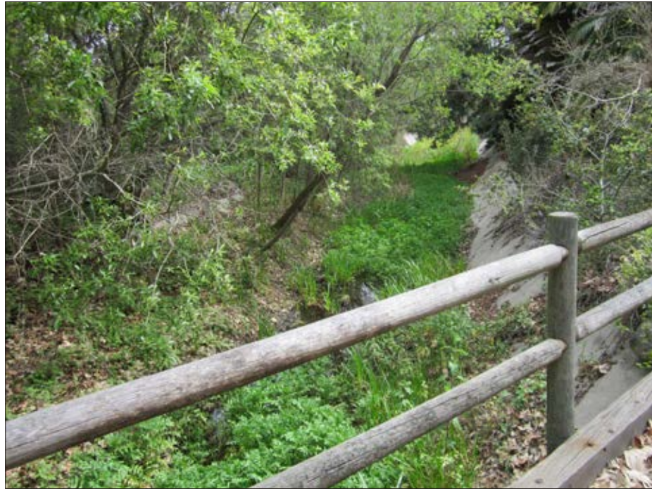
Photo 1: Downstream of beach access road bridge
