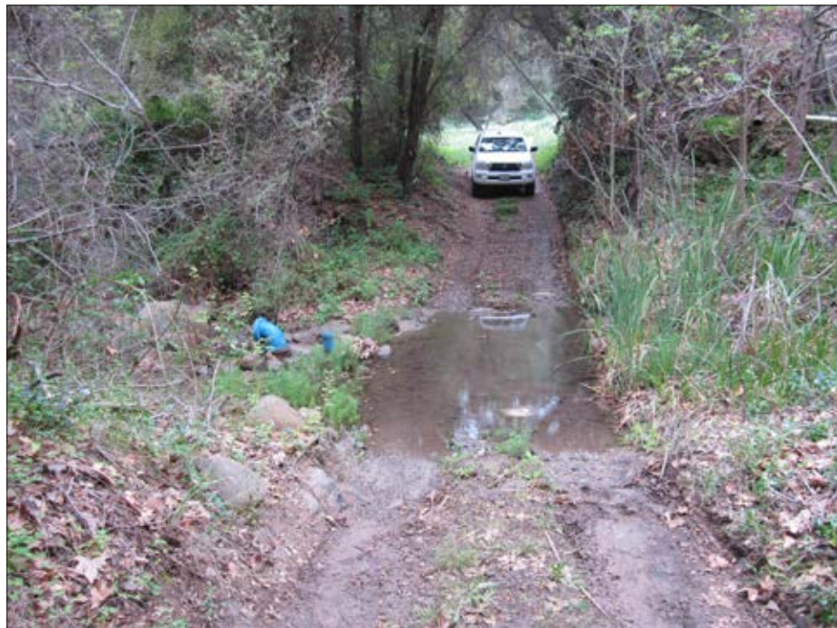
Photo 4: View of unpaved low water crossing looking west
