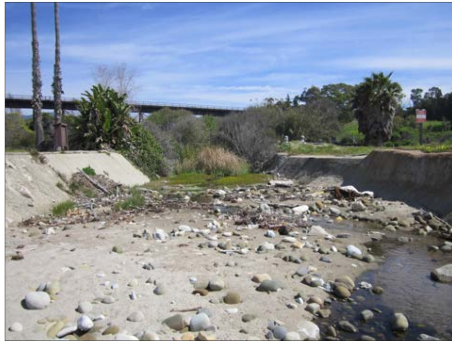
Photo 2: Concrete channel looking northeast
