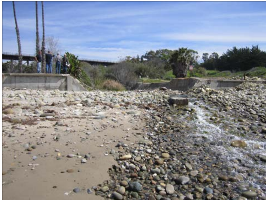
Photo 1: Beach outfall looking northeast
