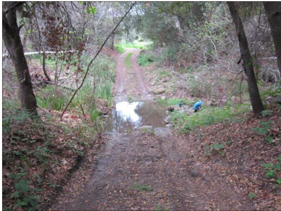
Photo 1: View of unpaved low water crossing looking east
