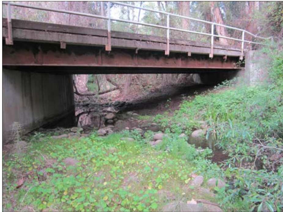
Photo 4: Underneath La Casa Grande Bridge
