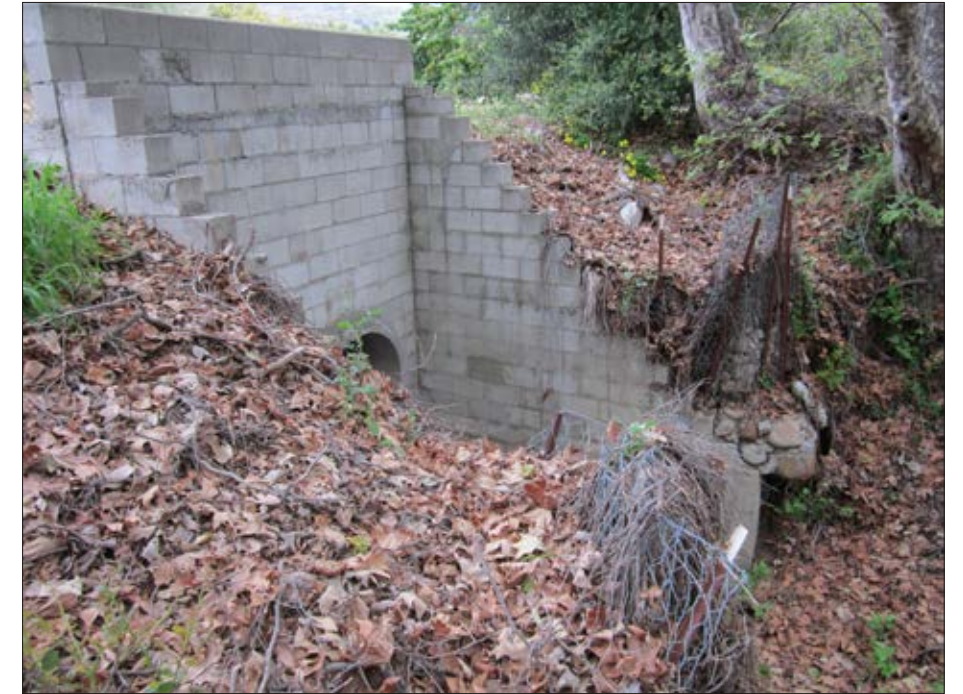
Photo 3: View of agriculture drain structure/culvert on east side of access road
