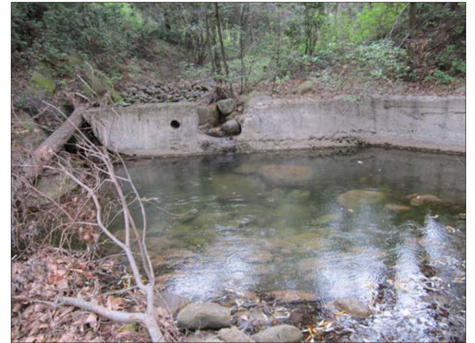
Photo 3: View of old flood gate and wall structure looking north
