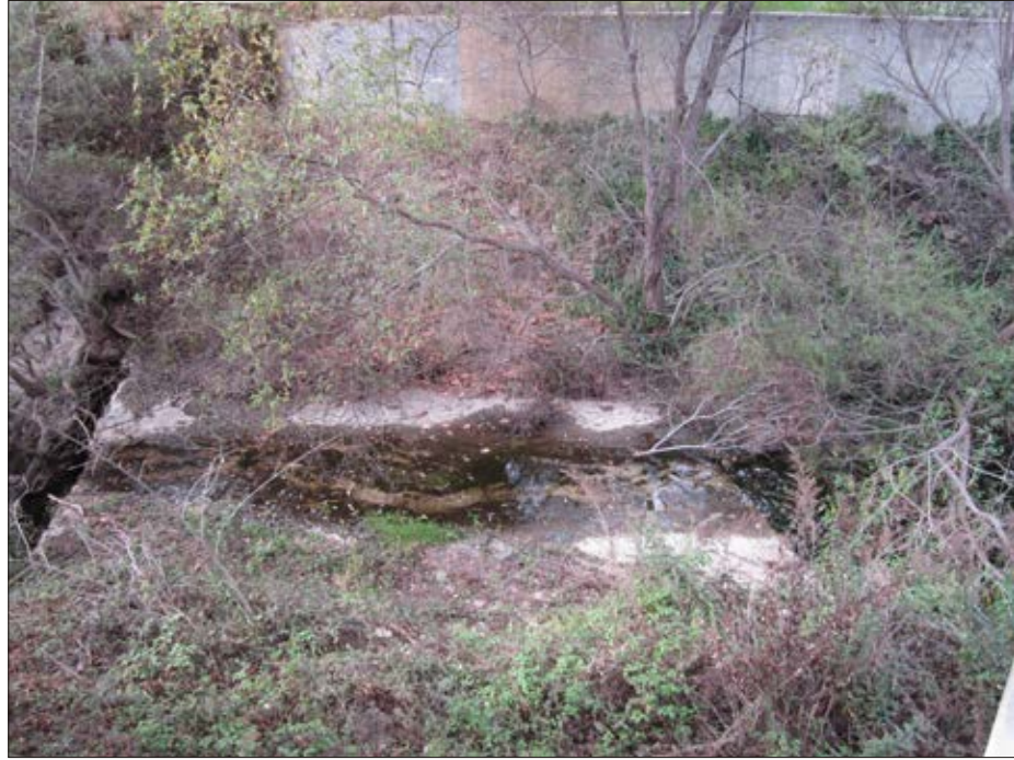
Photo 1: Hwy 101 bridge concrete paving and drop structure
