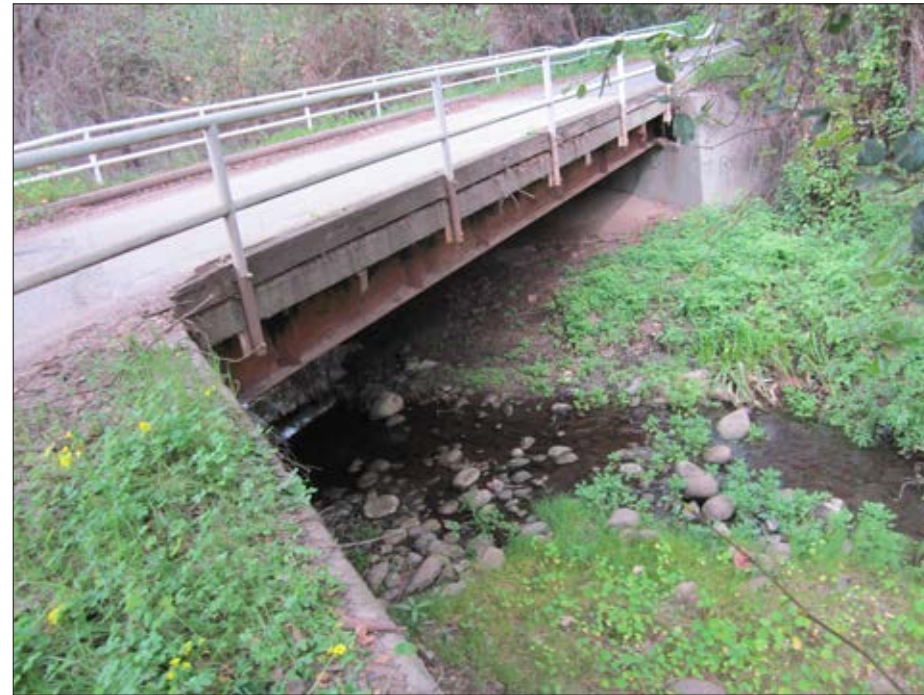
Photo 5: Looking into creek at upstream side of La Casa Grande Bridge
