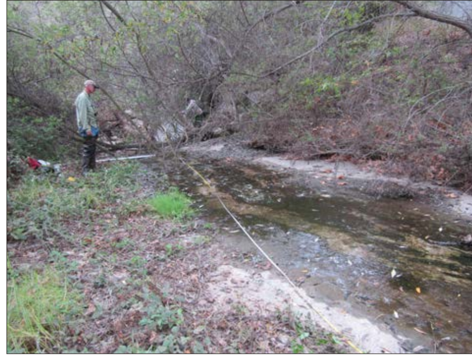
Photo 2: Old concrete paving under bridge looking south towards drop structure
