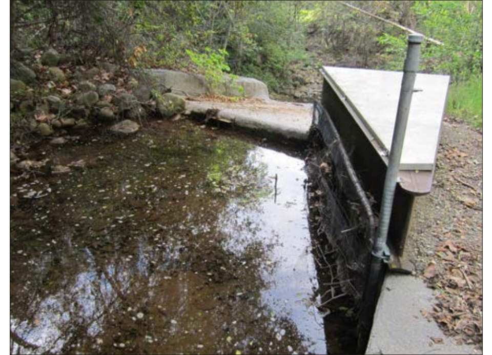
Photo 3: View of weir structure and pool looking south
