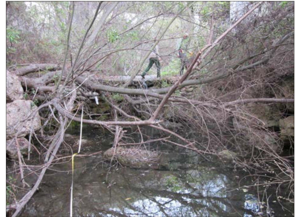
Photo 6: View looking north along lower pool towards spillway of drop structure
