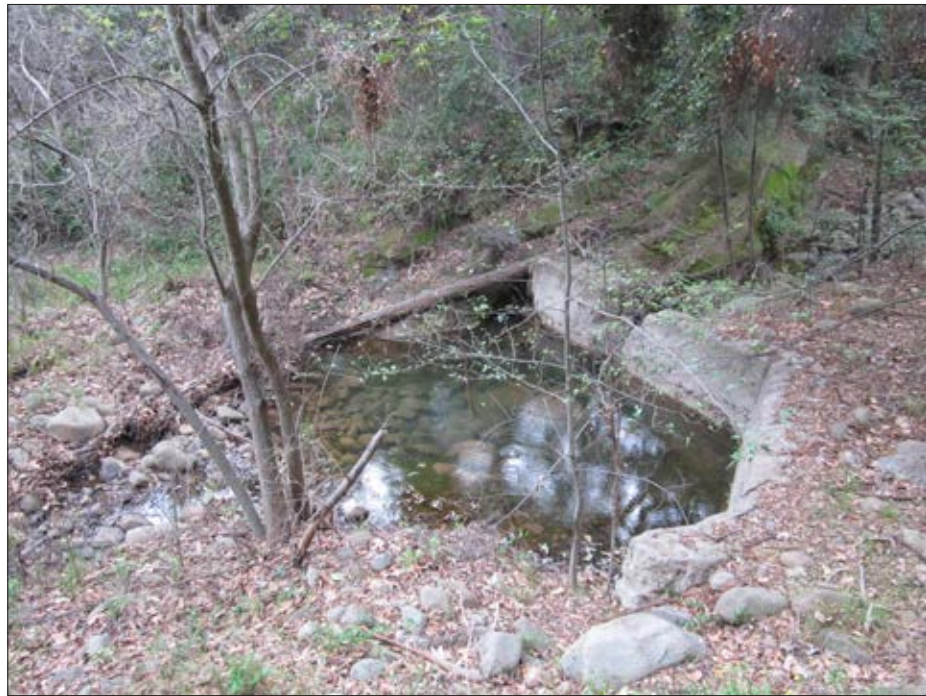
Photo 1: View of old flood gate and wall structure looking northwest
