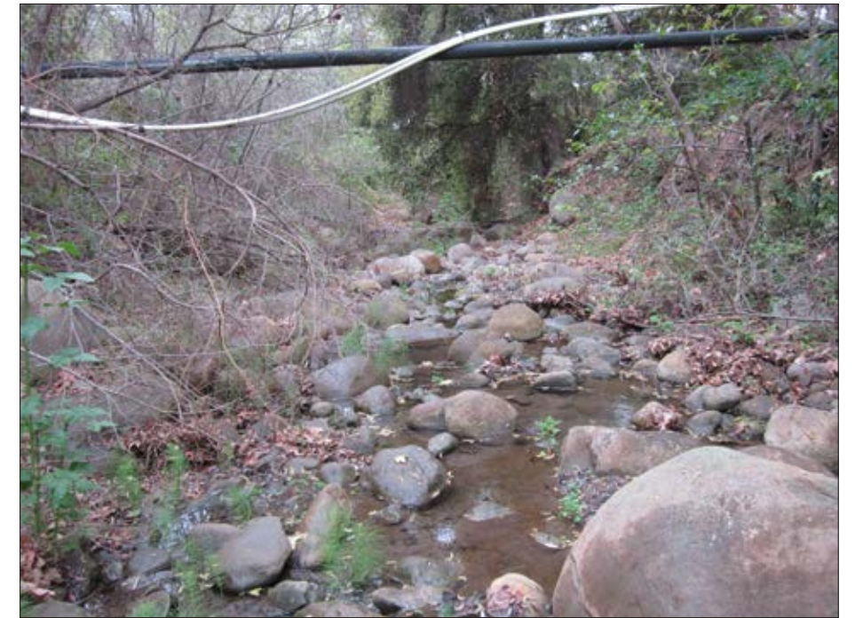
Photo 3: View of unpaved low water crossing looking downstream (south)
