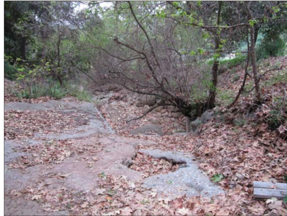
Photo 2: View of paved low water crossing looking south
