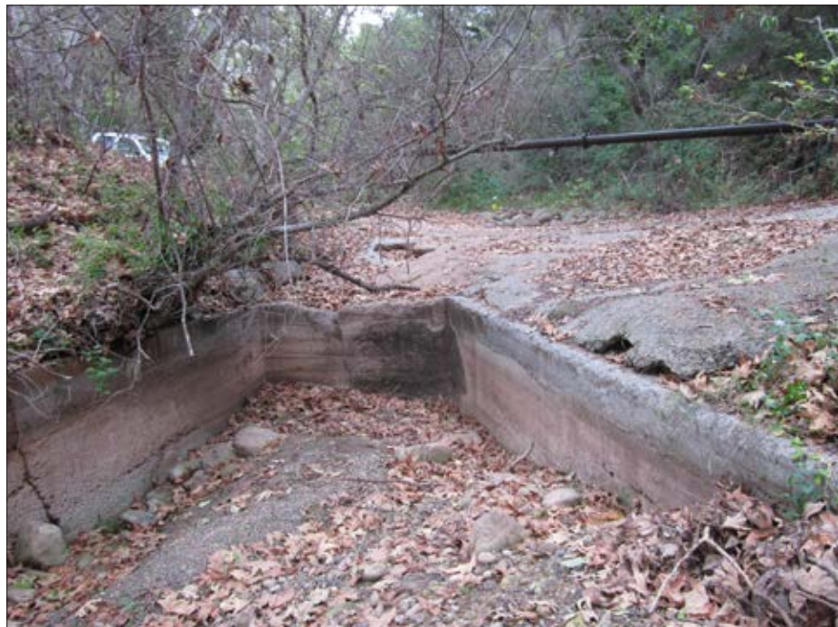
Photo 4: View of paved low water crossing & grade control crossing looking north
