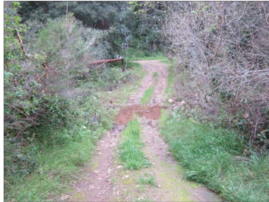
Photo 5: View of low water crossing looking west
