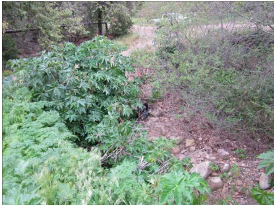
Photo 4: View of creek downstream of culvert crossing looking south
