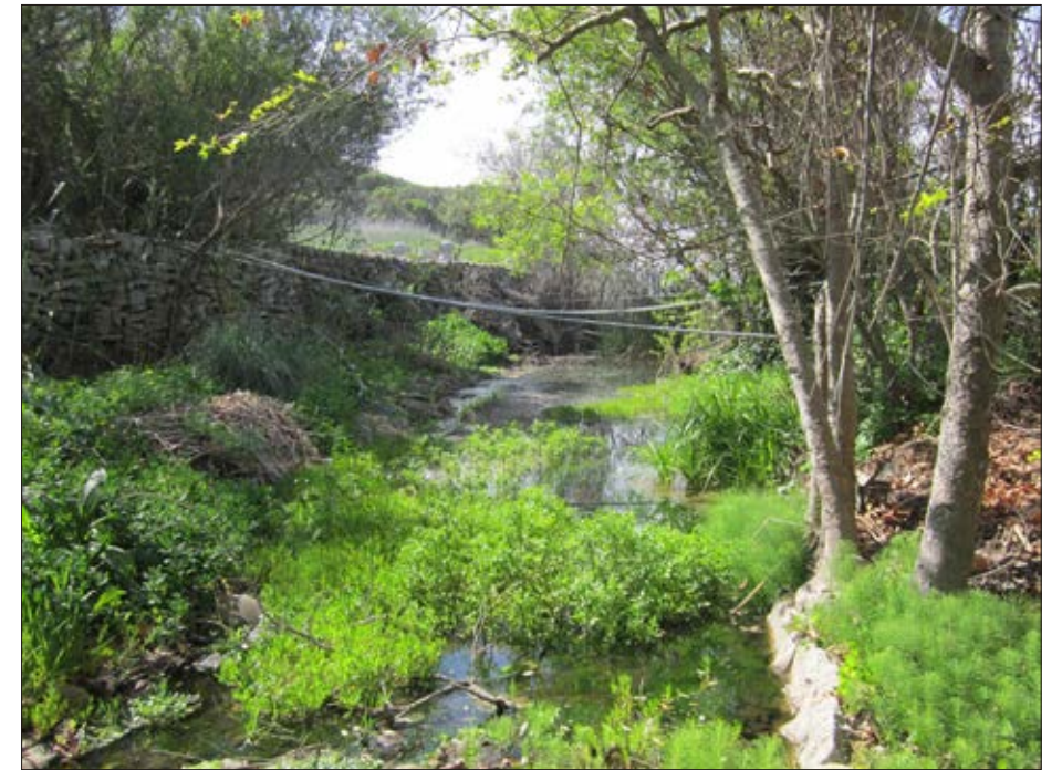
Photo 3: Creek channel bank protection looking south
