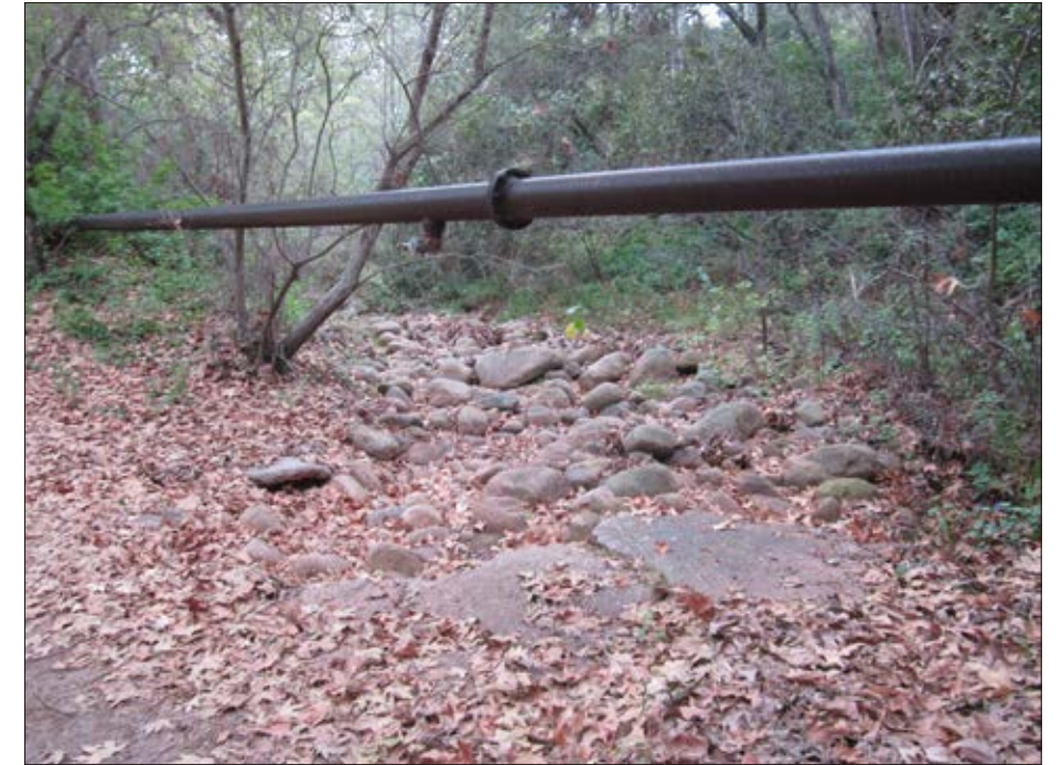
Photo 3: View of paved low water crossing looking north
