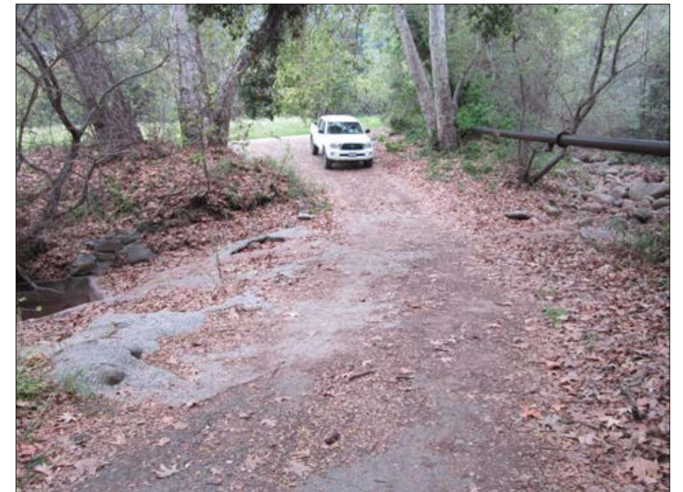
Photo 6: View of paved low water crossing looking west
