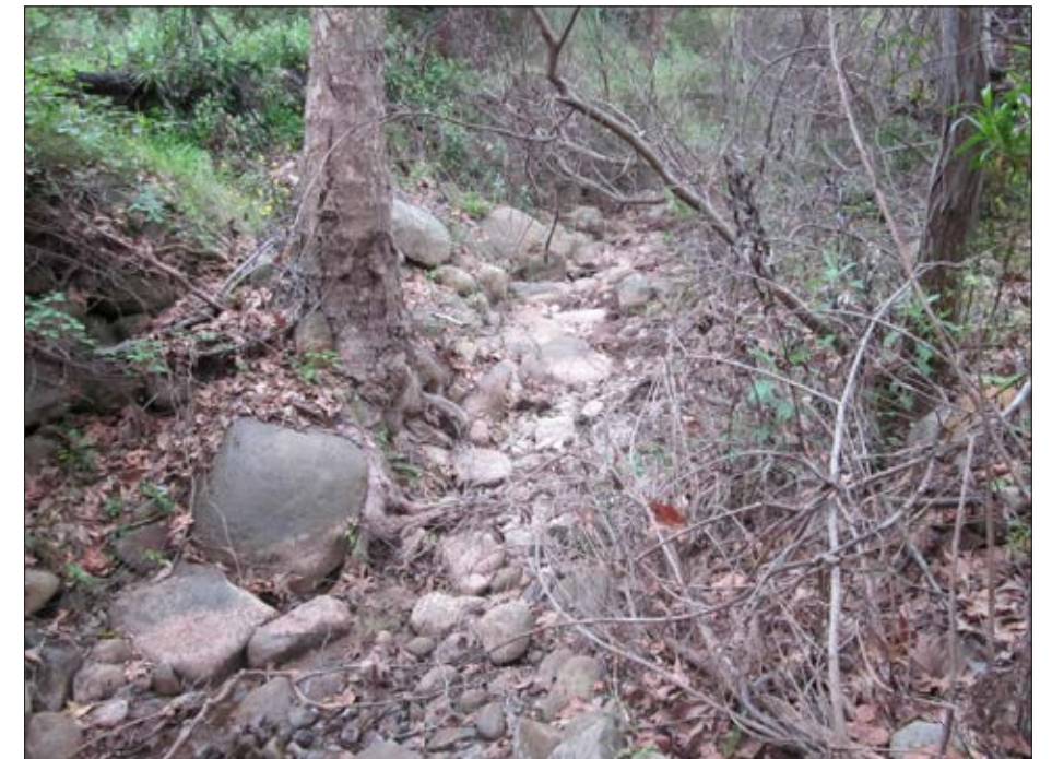
Photo 6: View of creek downstream of old flood gate and wall structure
