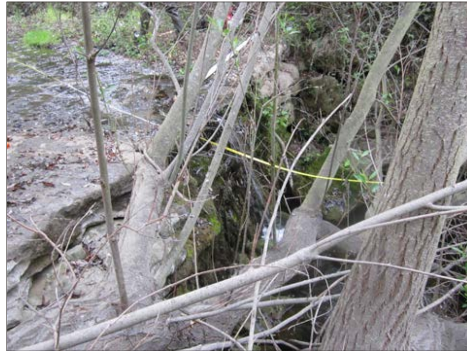
Photo 5: View looking east at spillway of drop structure
