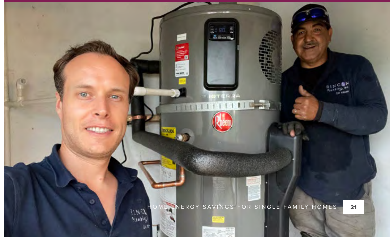
Zev and his employee, Jesus, after a successful 65 gallon HPWH installation.
