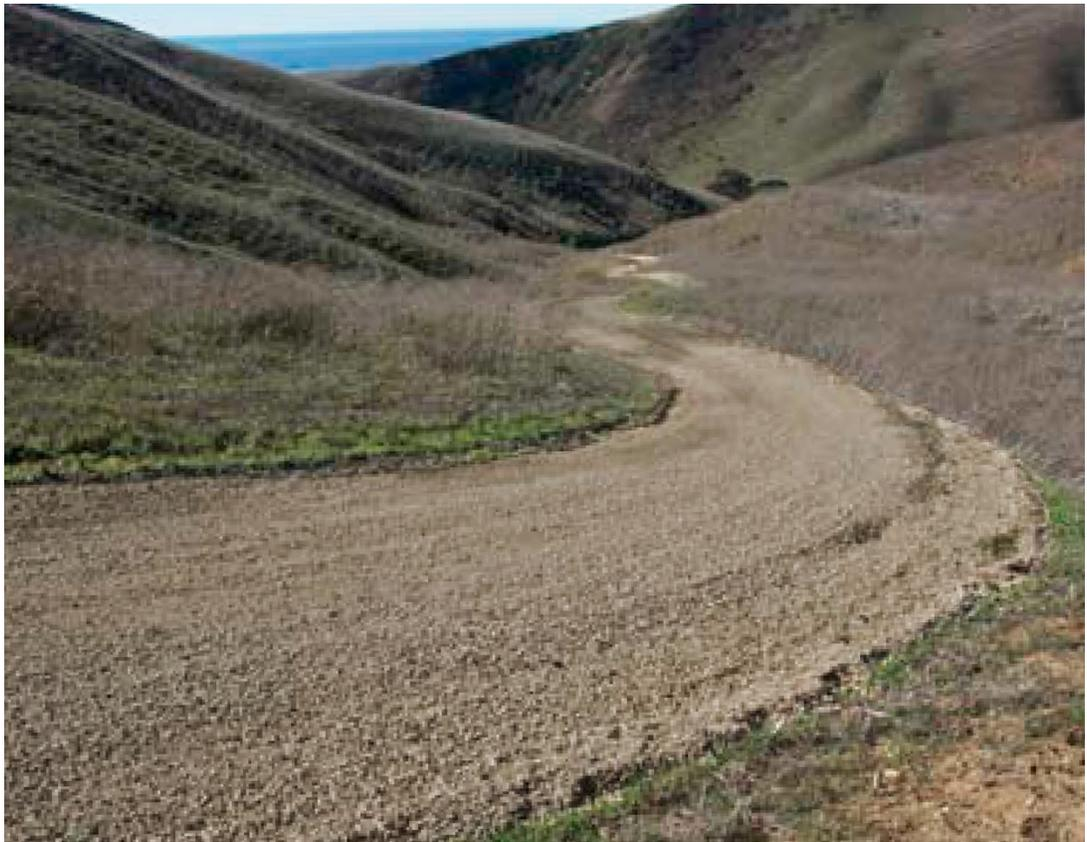
*Shale and permeable base roads are encouraged as they are compatible with wildlife corridors and animal husbandry, and are visually unobtrusive as in this case. Roads located in natural draws are encouraged.*
