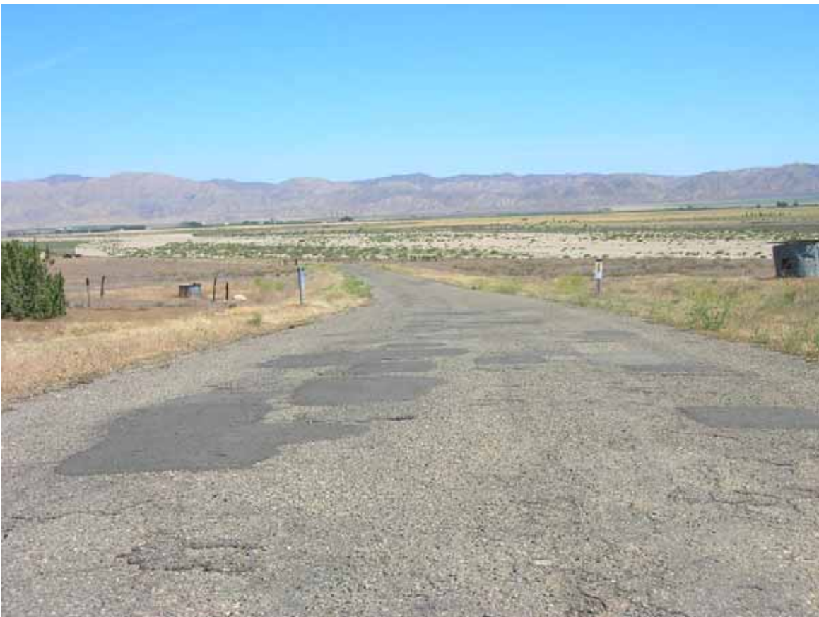
Santa Barbara Canyon Road, Cuyama
