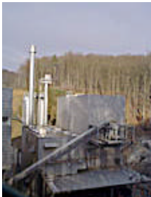
EVA energy plant at Aßlar
