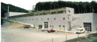
Herhof Aßlar Stabilate and Energy Plant
