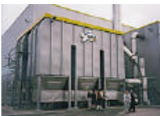
LARA system at Rennerod
