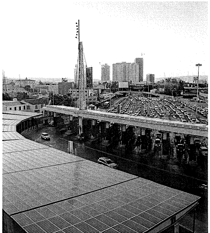
↑ General Services Administration – San Ysidro Land Port of Entry Phase II, a Turner & Townsend Heery Project
