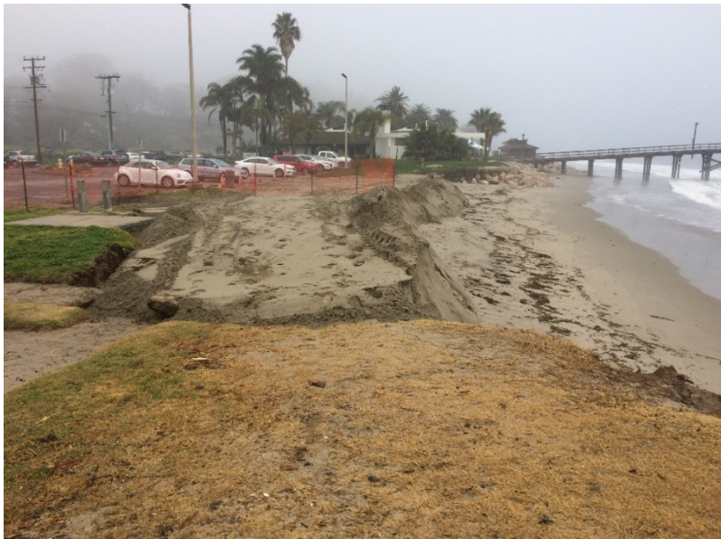
Eroded Central Park - Berm West of Restaurant January 2017
