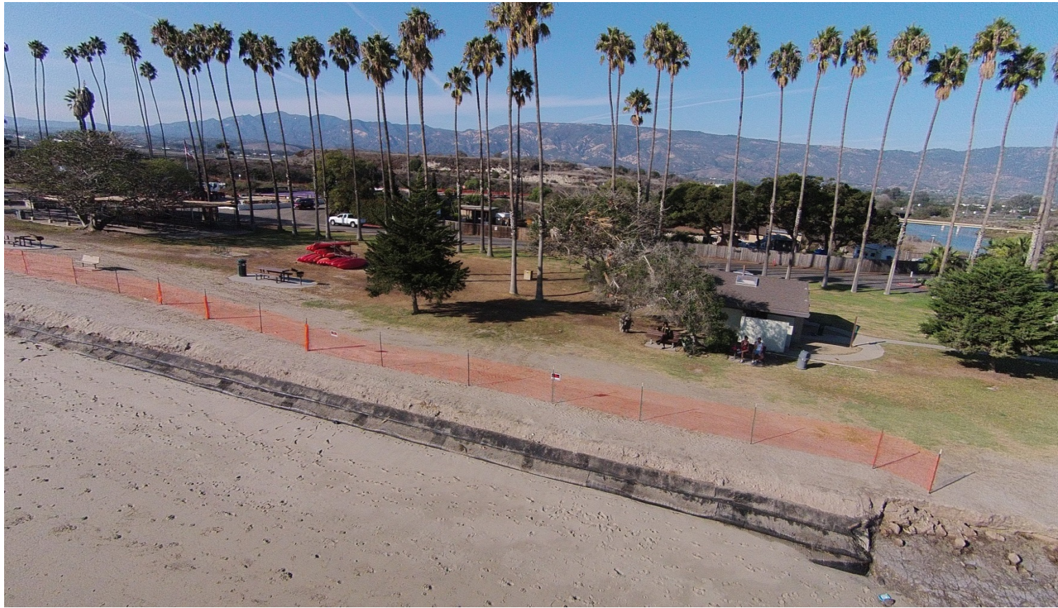
Geotextile Exposed From High Swells November 25, 2016
