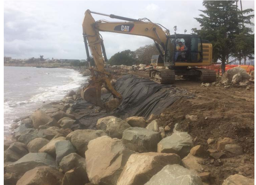
Revetment installation in front of Geotextile
