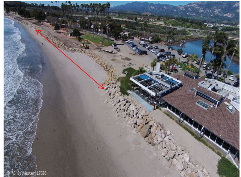
Added 948 foot Revetment - 2017
