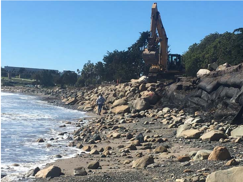
Revetment installation in front of Geotextile
