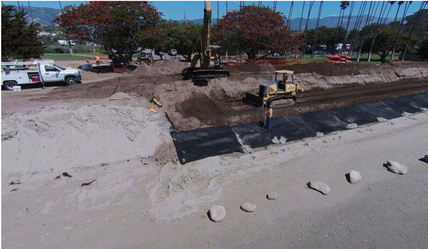
Installation of Geotextile April 2016 Cost $350,000
