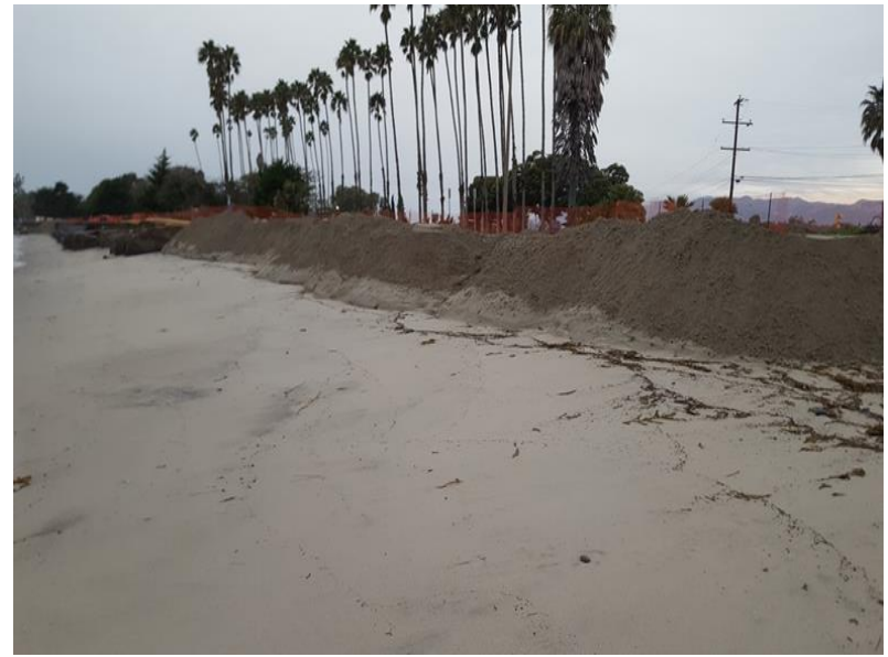
Eroded Central Park – Berm January 2017
