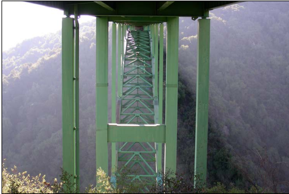
Photograph 3: Cold Spring Canyon Bridge substructure, camera facing southeast, 2/14/07.
