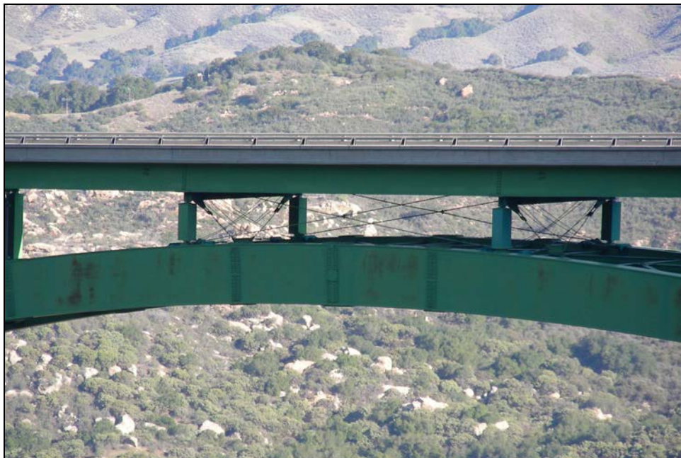
Photograph 4: Cold Spring Canyon Bridge arch apex, camera facing northeast, 2/14/07.
