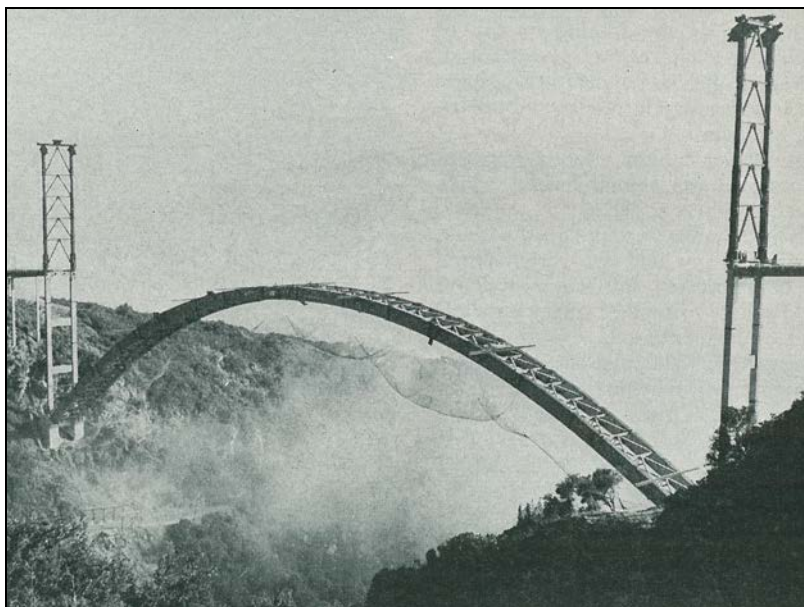
Photograph 6: Cold Spring Canyon Bridge under construction, completion of arch. Caltrans Negative # 10182-4. 70
