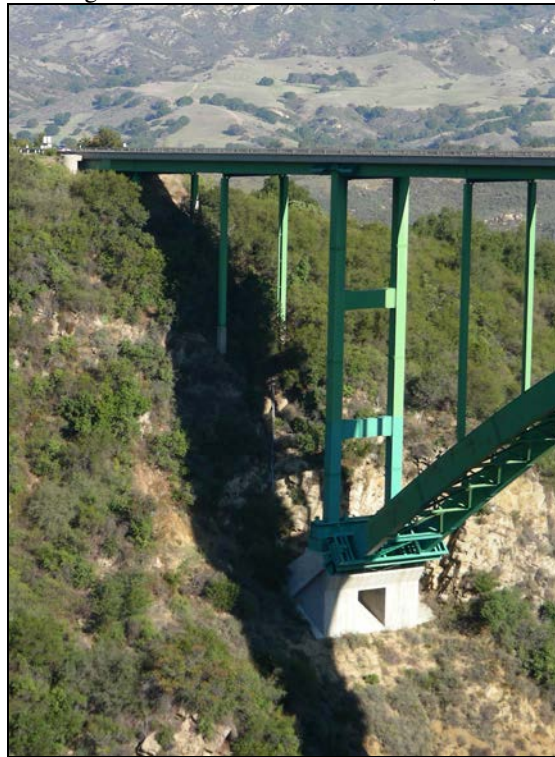
Photograph 10: Cold Spring Canyon Bridge west end, camera facing north, 2/14/07.
