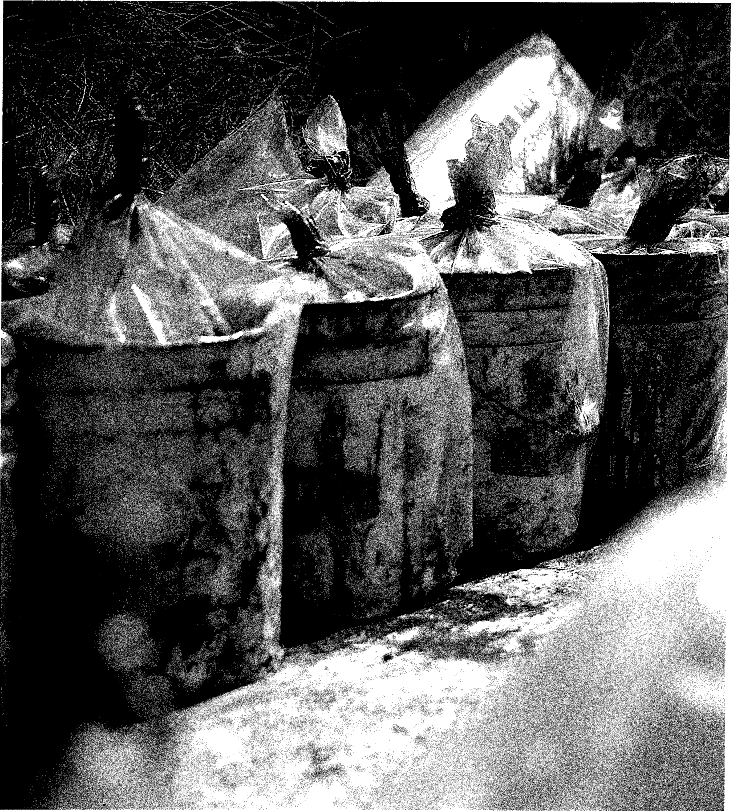
Buckets filled with oil-contaminated sand are lined up during a cleanup operation near Refugio State Beach on May 22, 2015, in Goleta, Calif.
