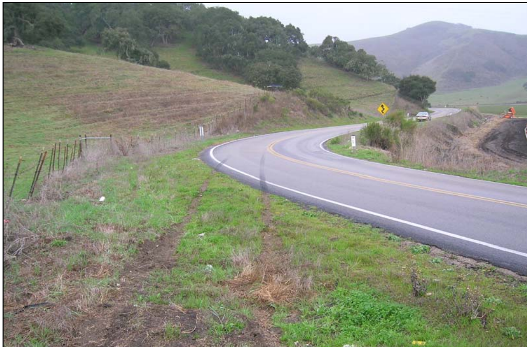
Harris Grade Road – Existing Conditions (Looking South)
