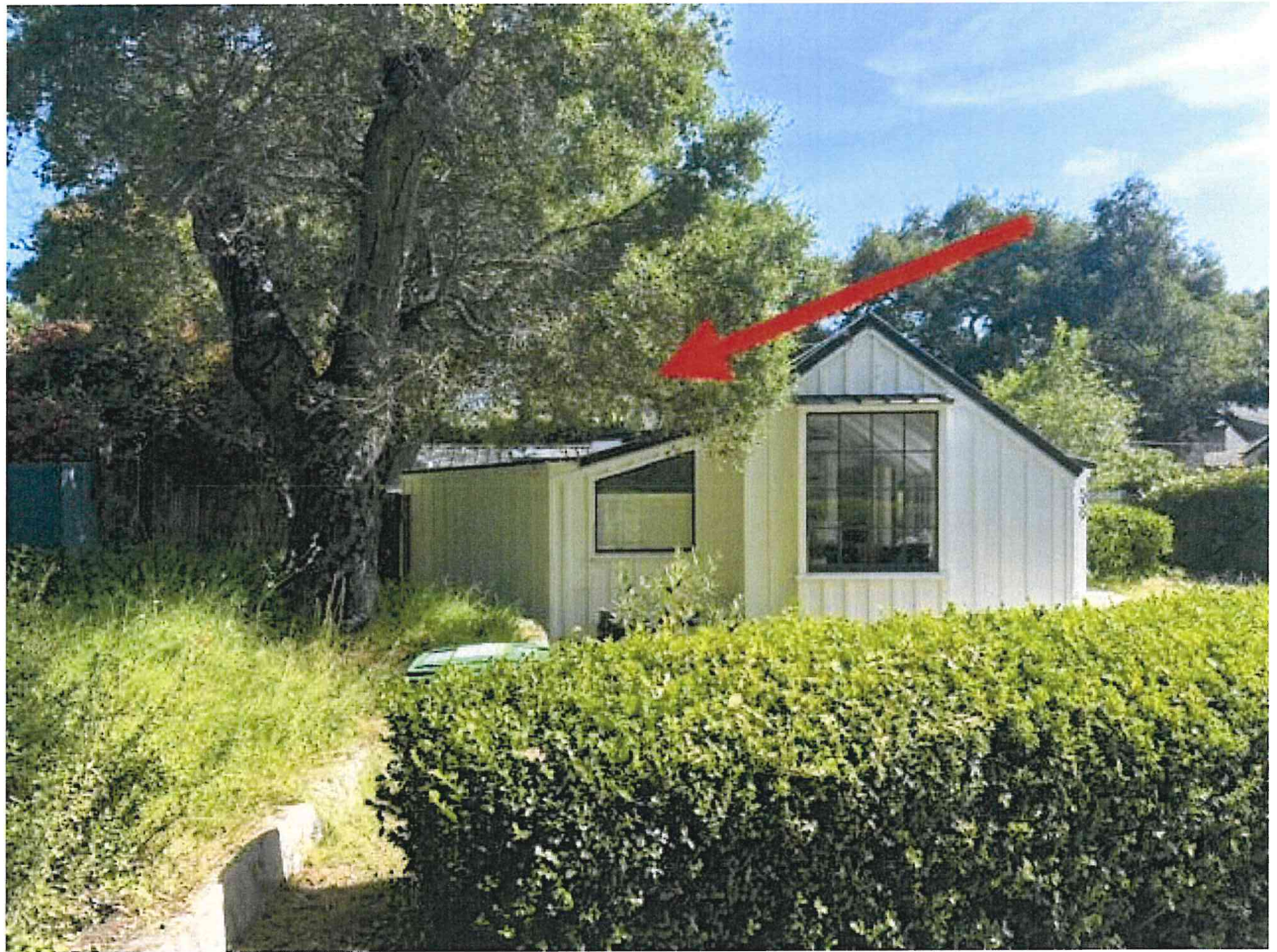
View of alterations from the street.
