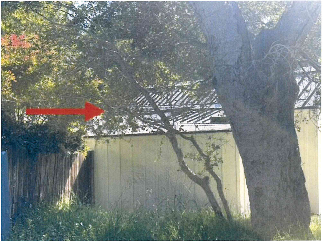
Raised dormer – view from Eastern elevation
