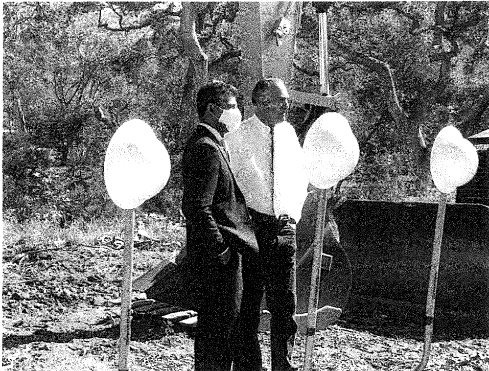
At Monday morning's groundbreaking ceremony, Supervisor Das Williams and Curtis Skene spoke of the efforts made to secure seven properties on Randall Road for a new Montecito debris basin along San Ysidro Creek. | Credit: Jean Yamamura
