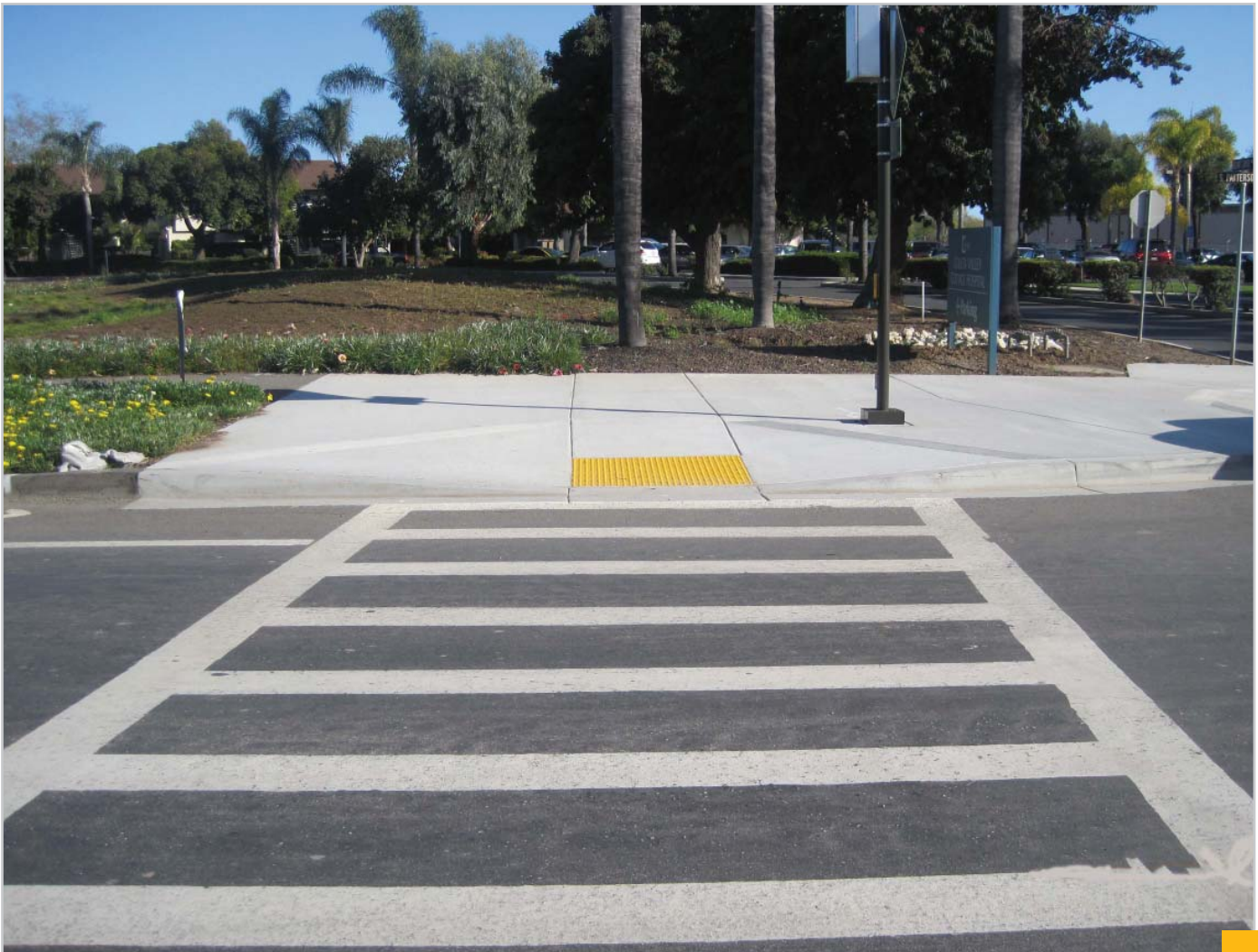
Photo Above: recently completed hardscape and ADA improvements
