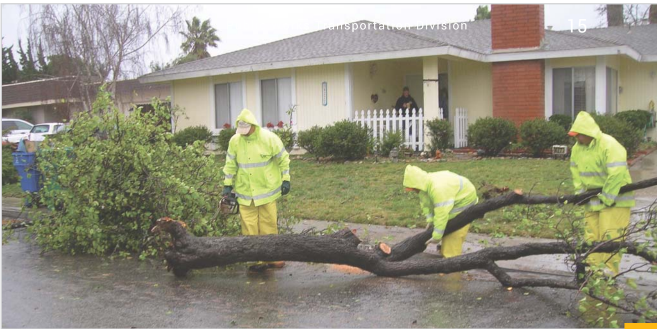
Photo: Maintenance crews perform emergency tree removal
