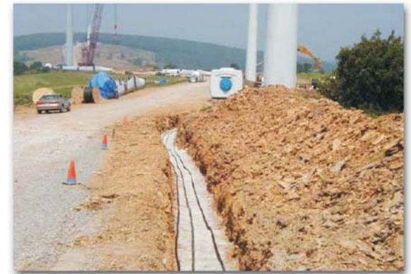
Inset C: Excavated trench for underground cables.
