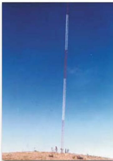
Inset G: Meteorological tower.
