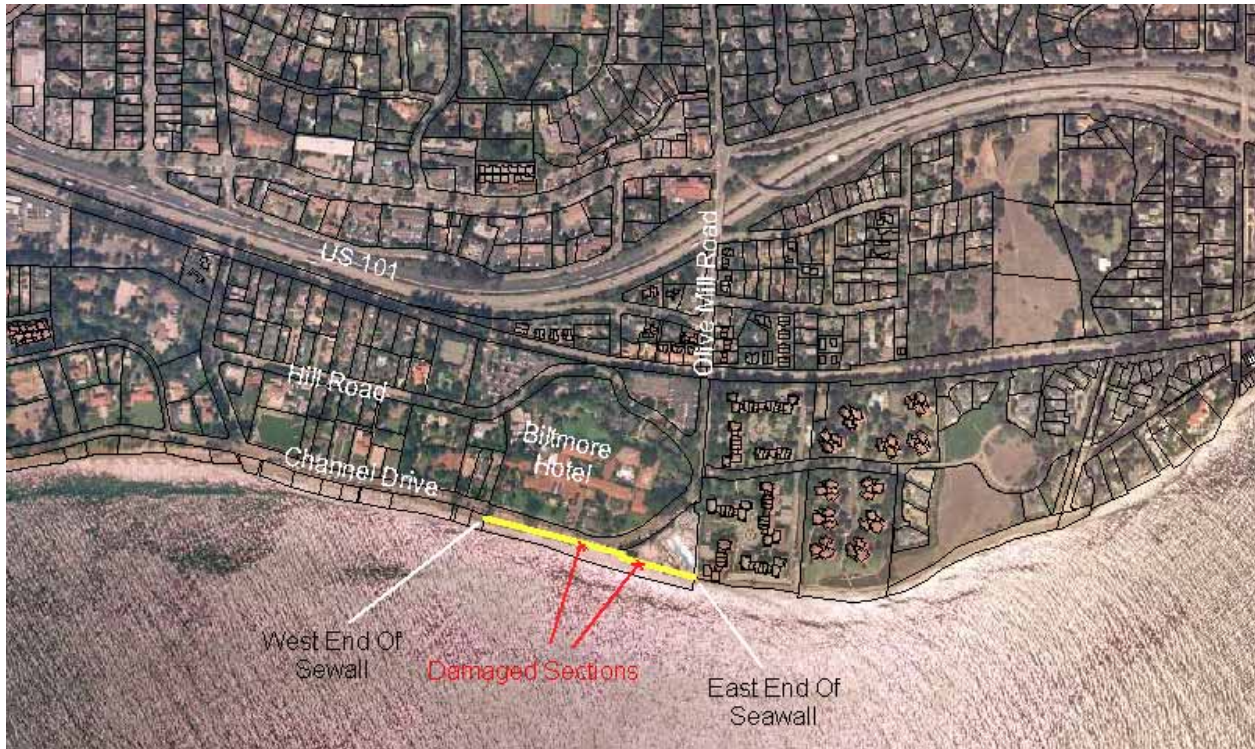
Figure 1: Biltmore/Coral Casino Seawall Failures
