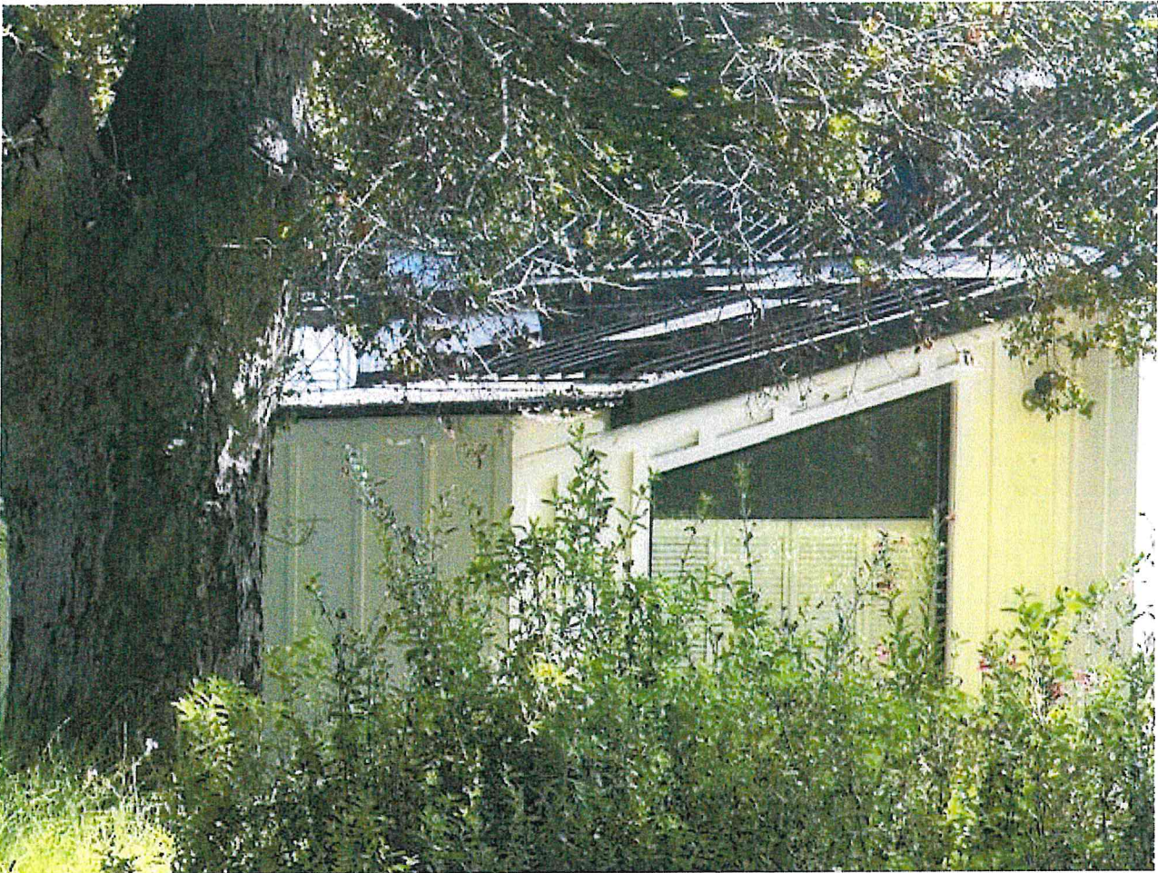
Raised dormer. Skylight was pre-existing.
