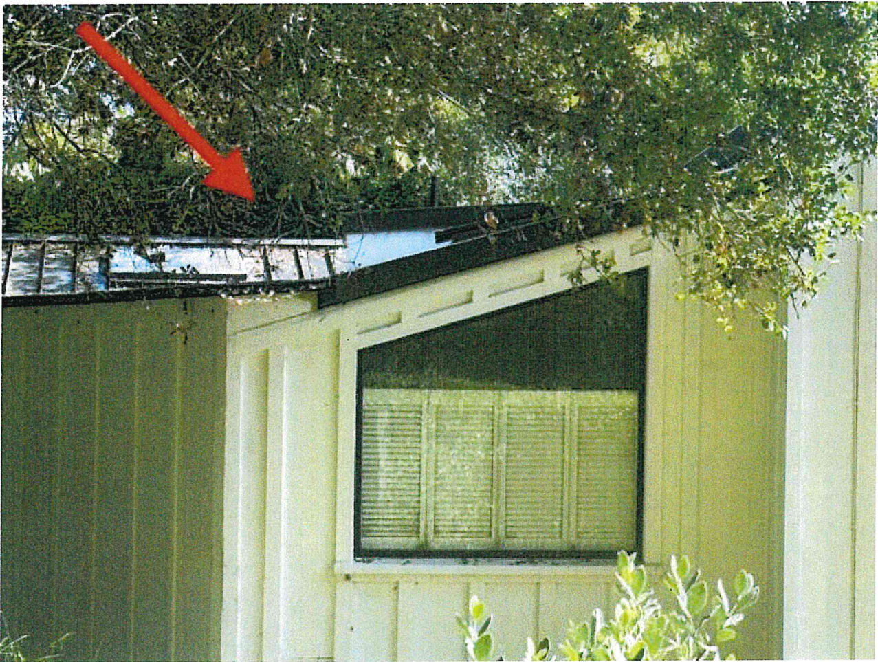
Here is the view of the raised dormer from the street.
