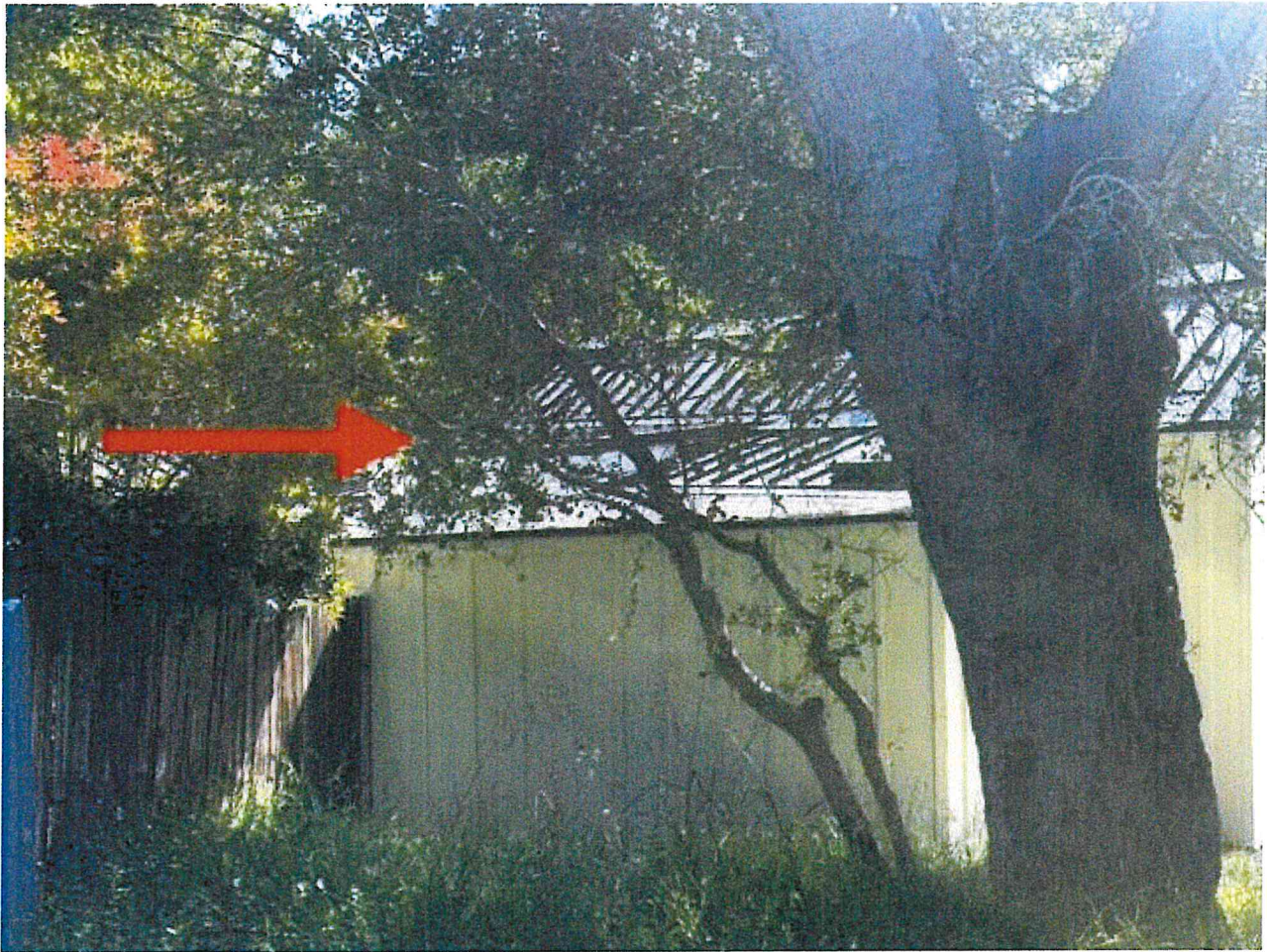
Raised dormer – view from Eastern elevation
