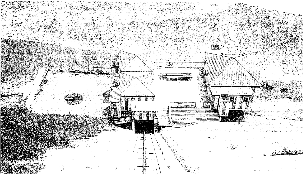
Beach cabana and built-up sand area behind rock wall at left, 1950s. Facing south
