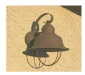
2. Partially Shielded. A fixture that may allow some light to pass through a semitranslucent barrier, and/or may allow visibility of the lamp from certain perspectives.
