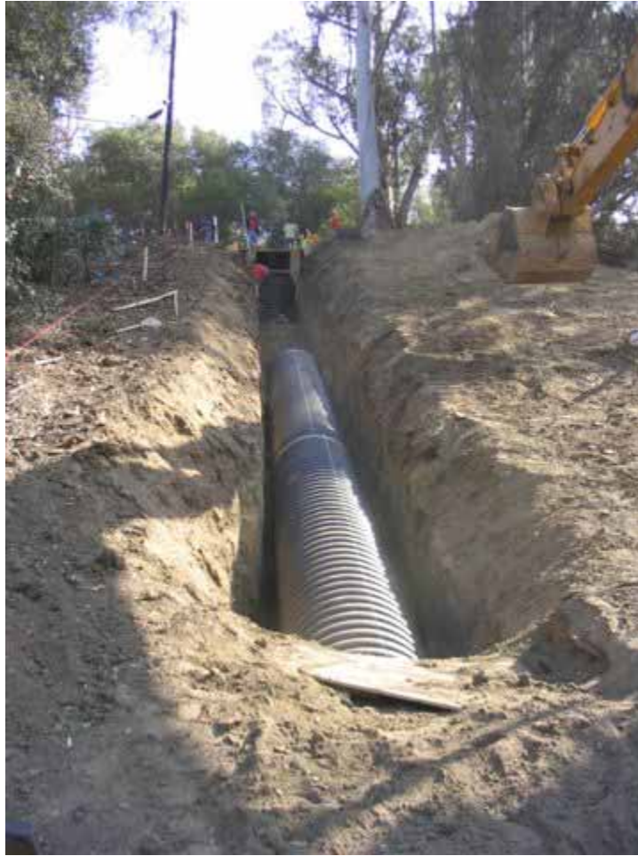
Via Rueda Interceptor Storm Drain Project Construction
