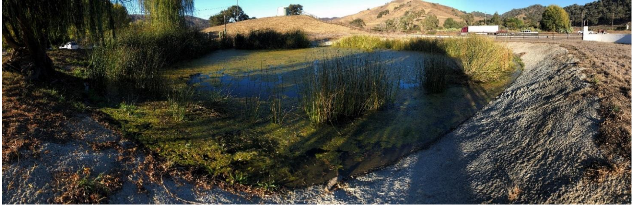
Concrete-lined agricultural reservoir used for irrigation located in southwest corner of property. View looking northeast. Reservoir is adjacent to US Highway 101 (upper right). Entrance driveway is to the right of the photo.
