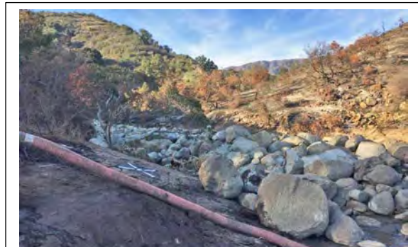
The Santa Monica Debris Basin was constructed as part of the Carpinteria Valley Watershed Project in the 1970s following a series of major flooding events that occurred along Santa Monica Creek.
