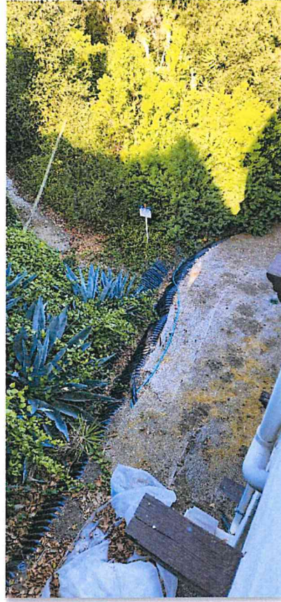
Photo 2: Exposed Panel Drain and HP
