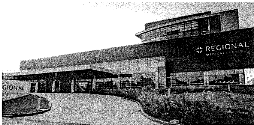
Regional Medical Center of San Jose, 4-Story Patient Wing Addition
