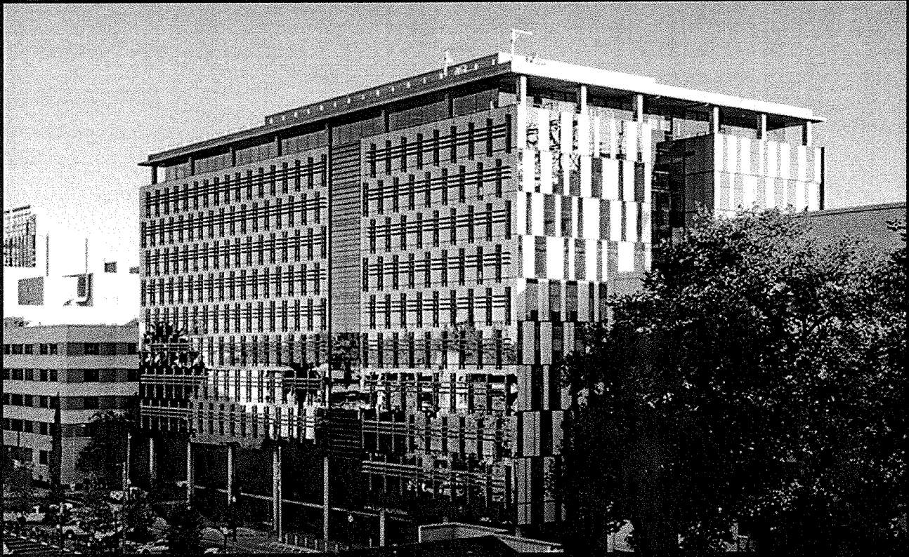
CA DGS, Clifford L. Allenby Office Building, Sacramento, CA
