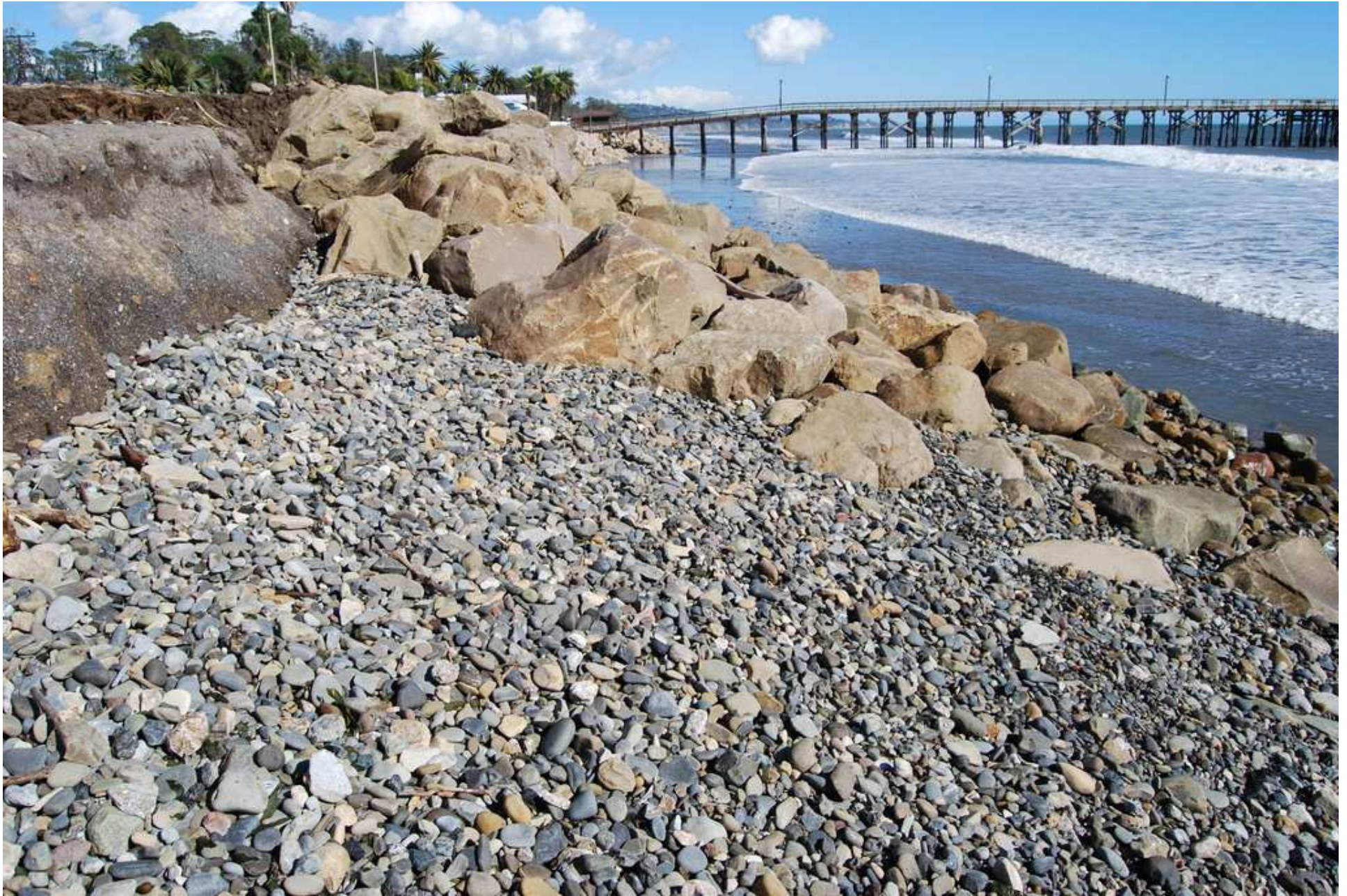
Natural wave-driven cobble berm approaches the volume of the new revetment.
