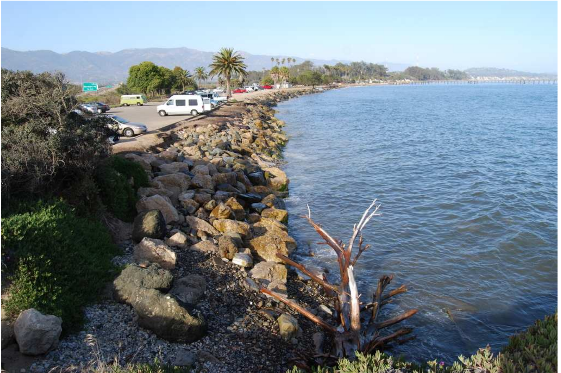
Goleta Beach, July 2017. West-end cobble berm protects access trail and vegetation from waves large enough to transport one-ton black boulders.
