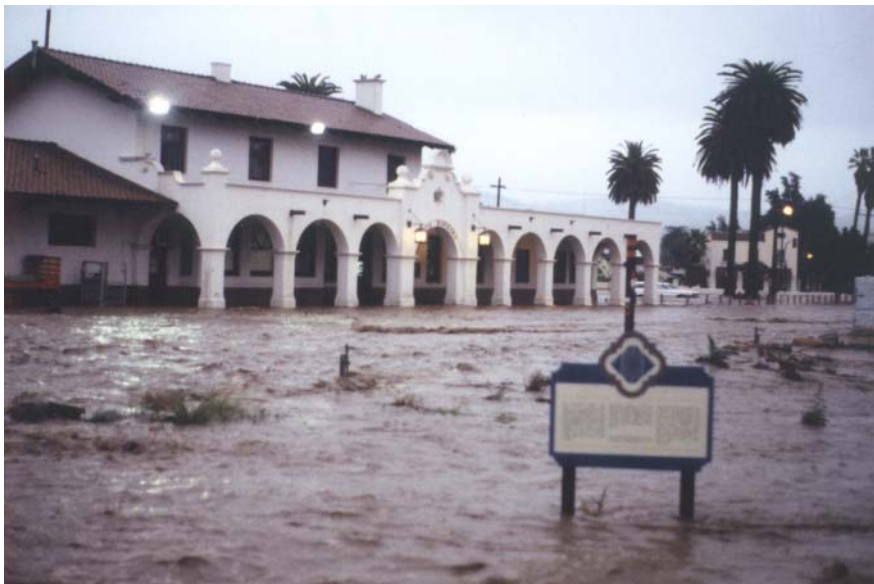
1995 Floods – Santa Barbara Train Station
