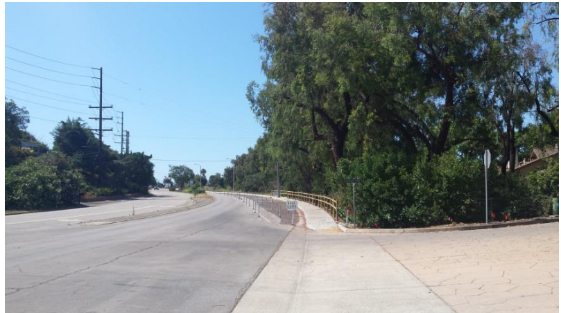
After - Patterson Avenue, looking south toward Tree Farm Development
