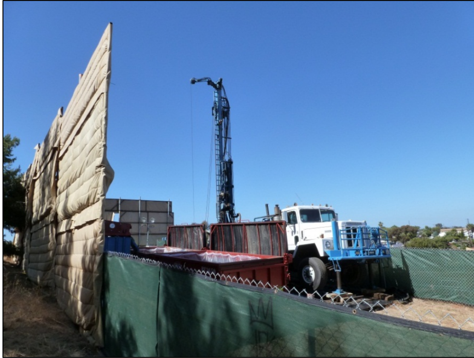
Figure 17 – Sample Temporary Construction Noise Barrier (URS, 2012)
