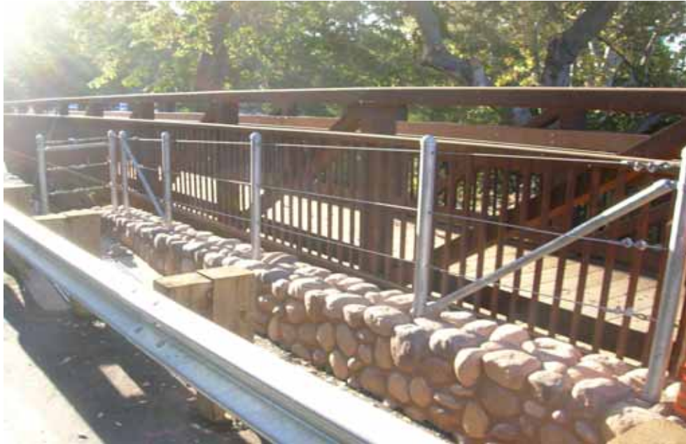
Montecito Pedestrian Bridge
