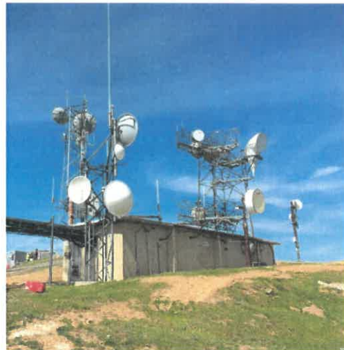
SBC small tower – by front left bldg corner
