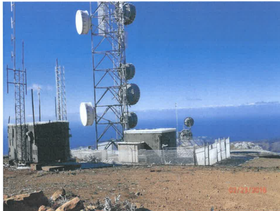
Facility #3 Touch Tel Corp (left), Facility #2 Freeport-McMoRan (right)
