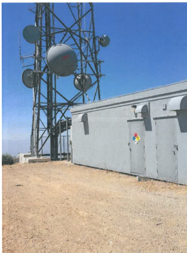
Facility #8 CA Highway Patrol/DGS
