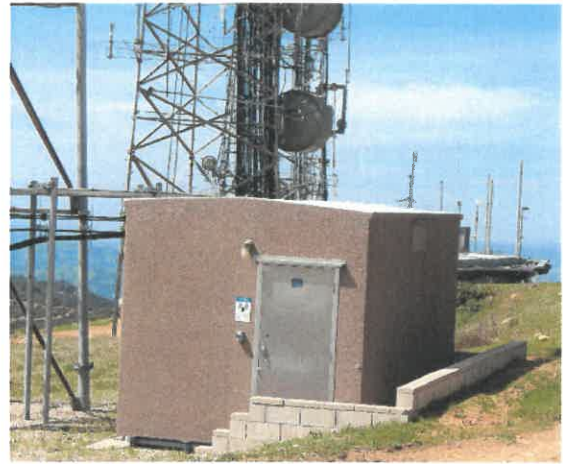
Facility #9 UPRR Co. vault
